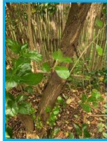
Tree 13: Trunk, decay and cracks throughout the trunk, supporting Tree 10. This tree may collapse, considerable risk to people and property.
