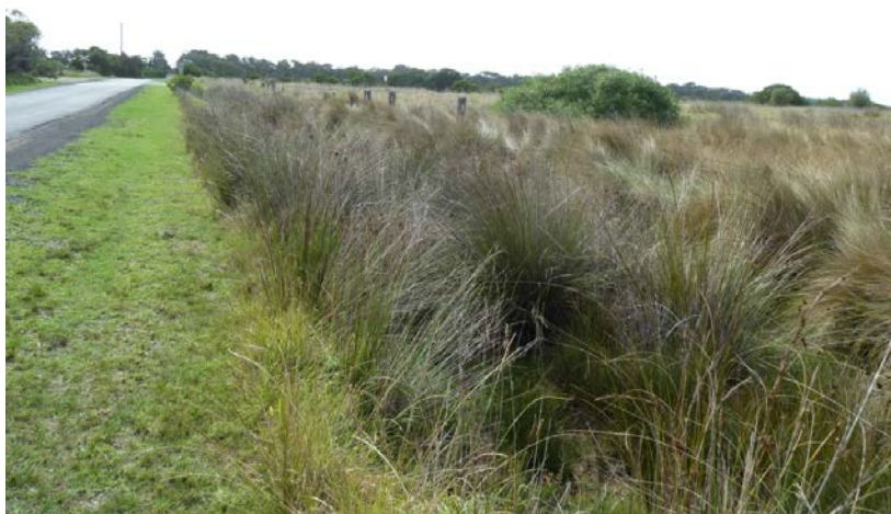
Figure 3 - Drainage channel adjoining the site along Murray Road
