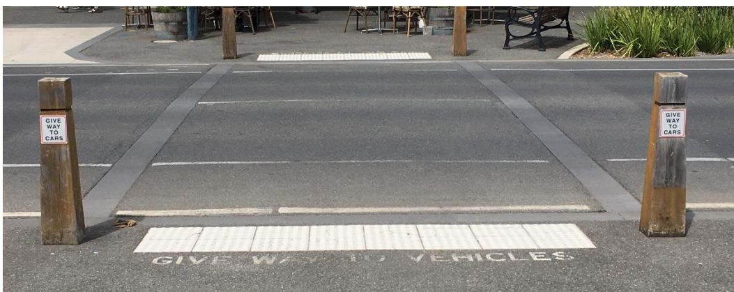
FIGURE 9: SIGNS AND LINEMARKING AT CROSSING POINTS
