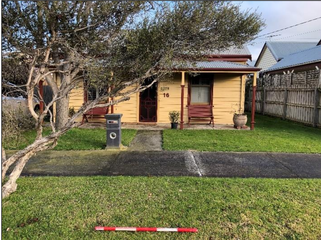
Plate 13: 16 Bay Street front view
