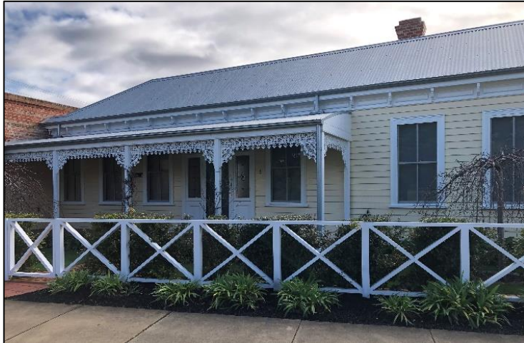
Plate 115: 8 Wharf Street front view
