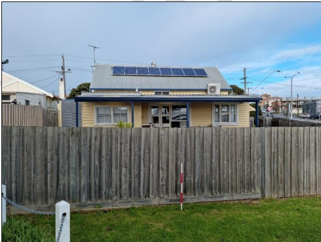
Plate 157: 46 Wharf Street rear view
