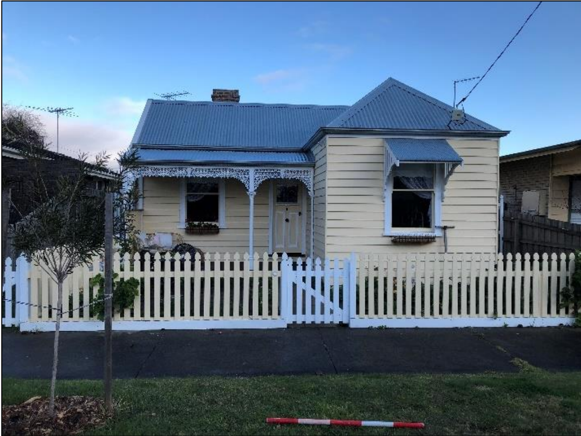
Plate 31: 8 Beach Street front view
