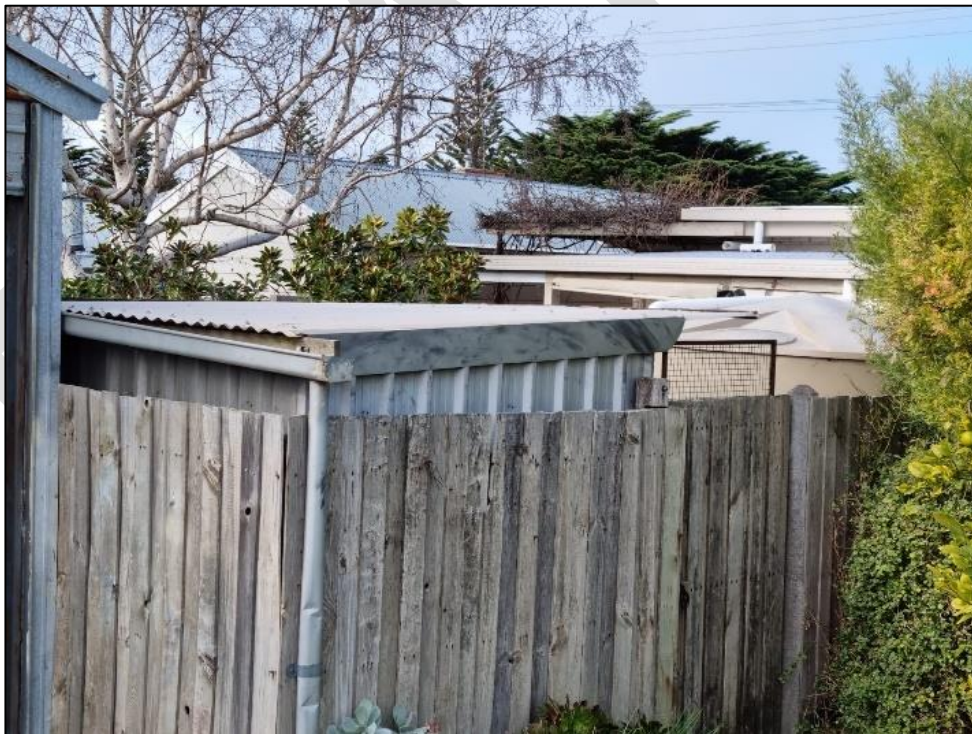
Plate 129: 18 Wharf Street rear view
