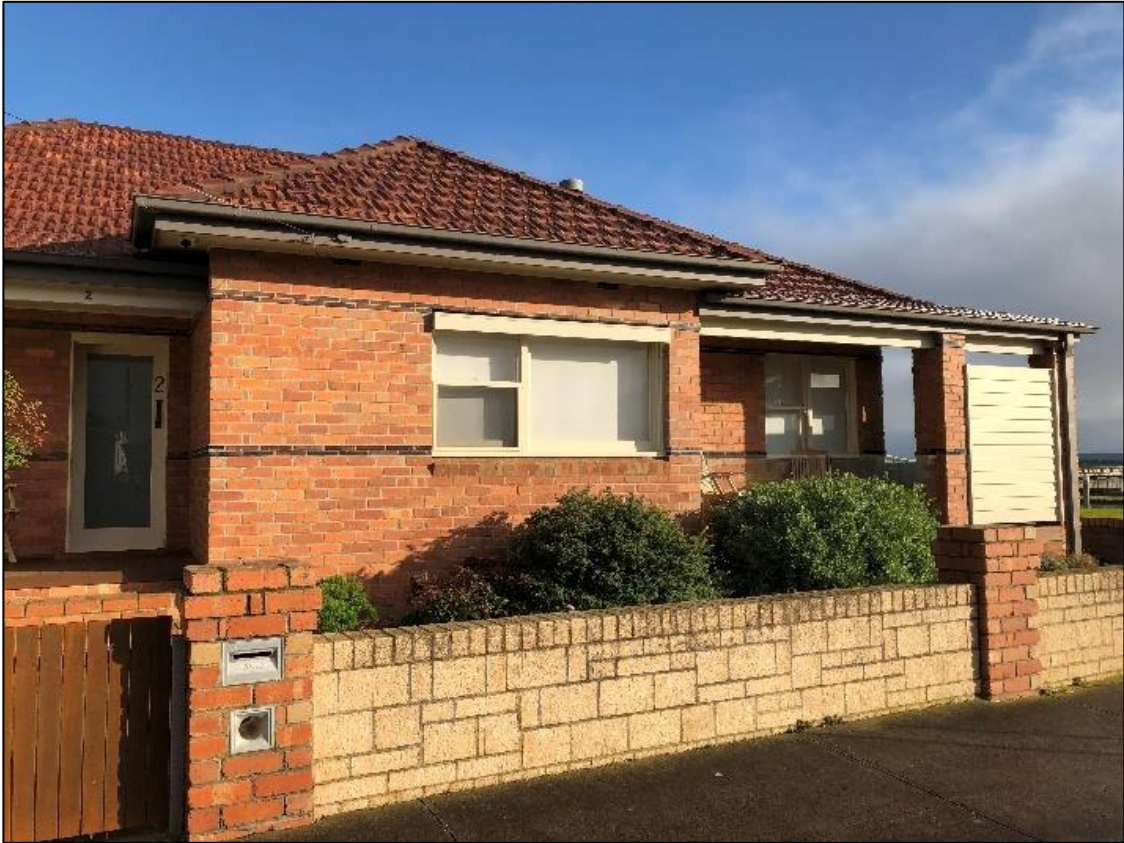
Plate 1: 2 Bay Street front view
