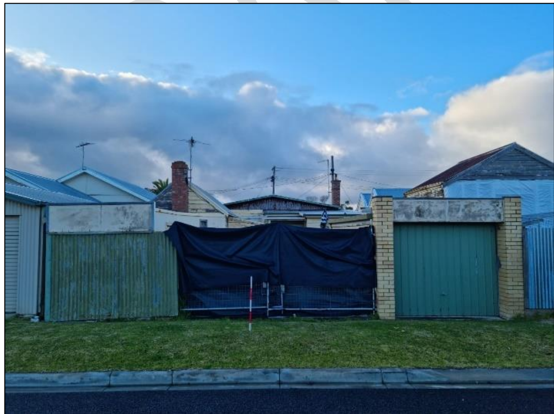
Plate 30: 6 Beach Street rear view with weatherboard Fishermans cottage to left ( brick chimney visible)
