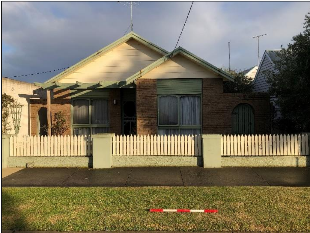
Plate 77: 36 Beach Street front view
