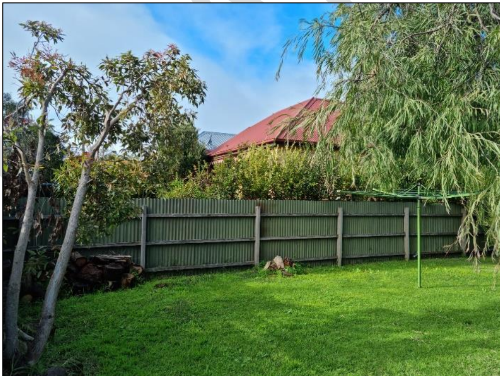
Plate 119: 10 Wharf Street rear view
