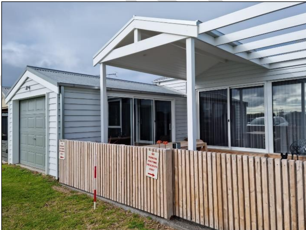
Plate 148: 38 Wharf Street rear view
