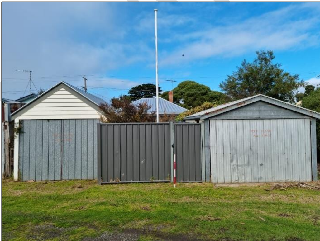
Plate 133: 22 Wharf Street rear view
