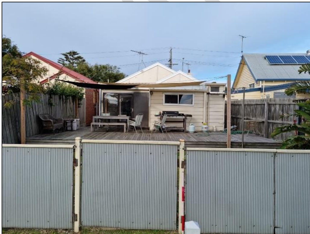
Plate 155: 44 Wharf Street rear view
