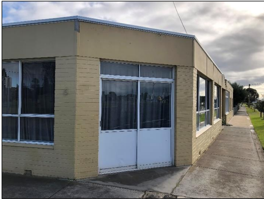
Plate 113: 6 Wharf Street side view
