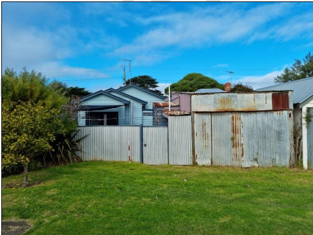
Plate 131: 20 Wharf Street rear view
