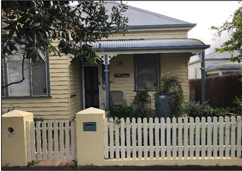
Plate 149: 40 Wharf Street front view
