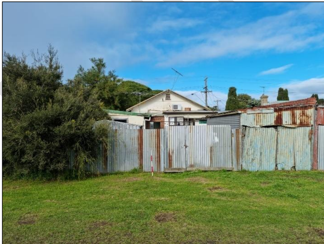
Plate 136: 26 Wharf Street rear view
