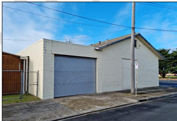
Plate 112: 4 Wharf Street side view
