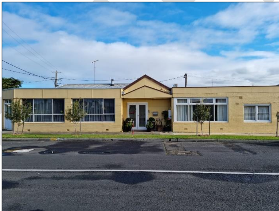
Plate 114: 6 Wharf Street front view
