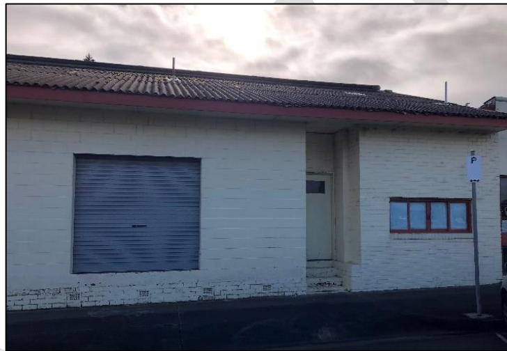
Plate 111: 4 Wharf Street front view
