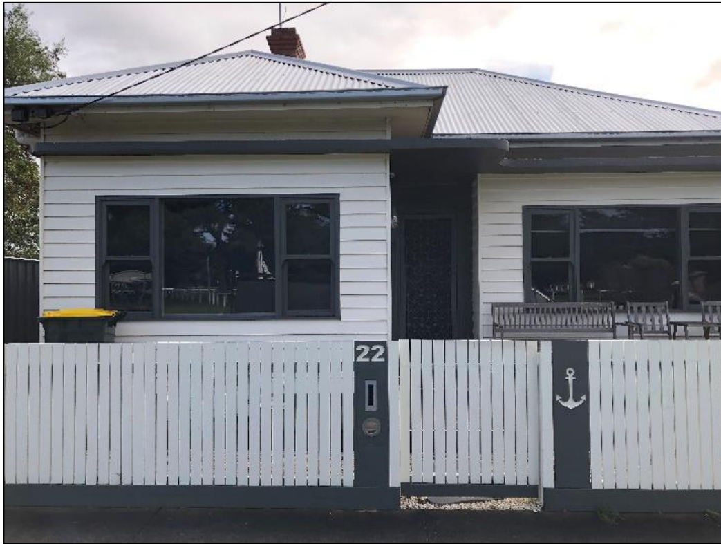
Plate 132: 22 Wharf Street front view
