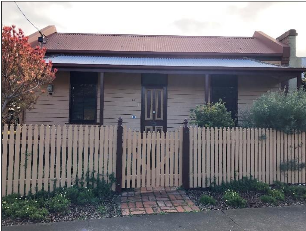
Plate 118: 10 Wharf Street front view
