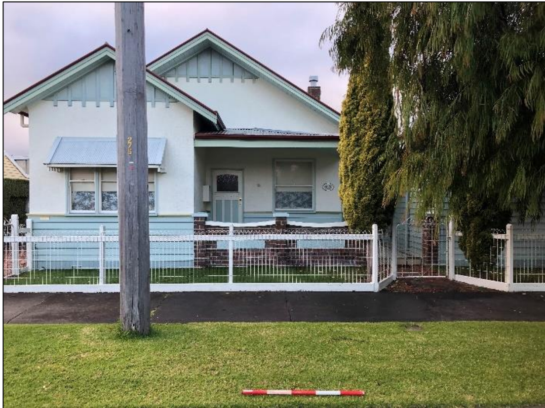
Plate 69: 31 Beach Street front view
