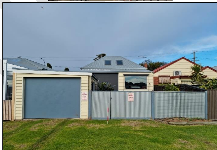
Plate 151: 40 Wharf Street rear view
