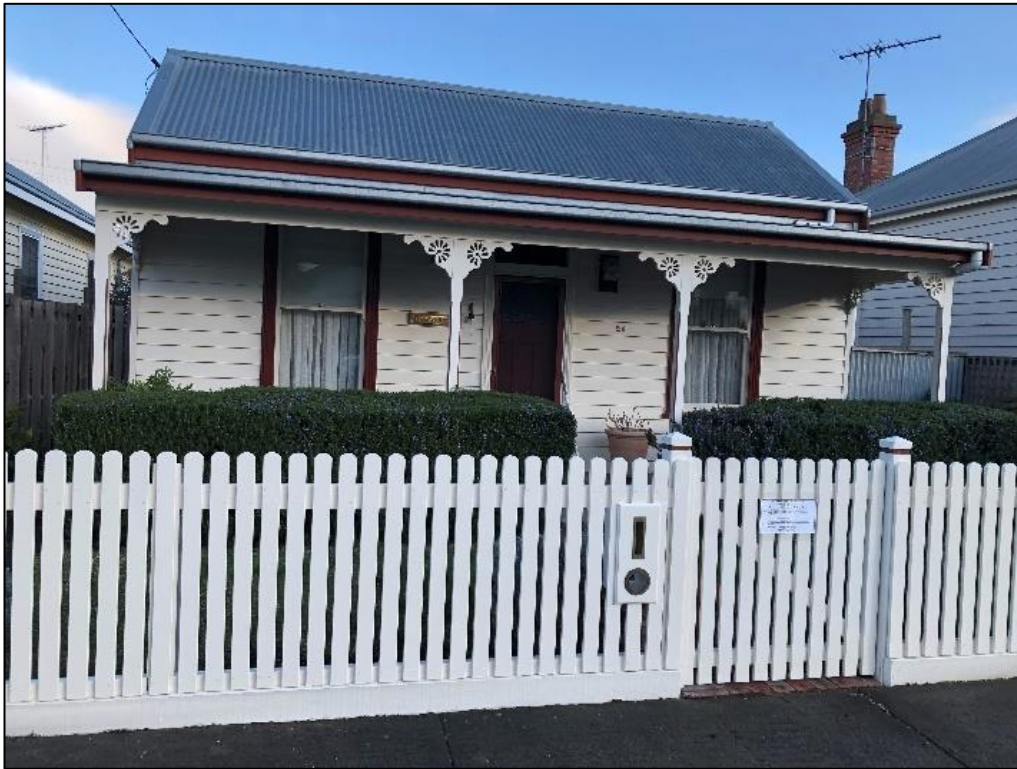
Plate 61: 26 Beach Street front view
