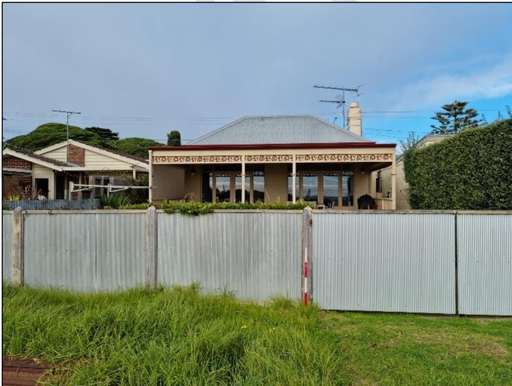
Plate 144: 34 Wharf Street rear view
