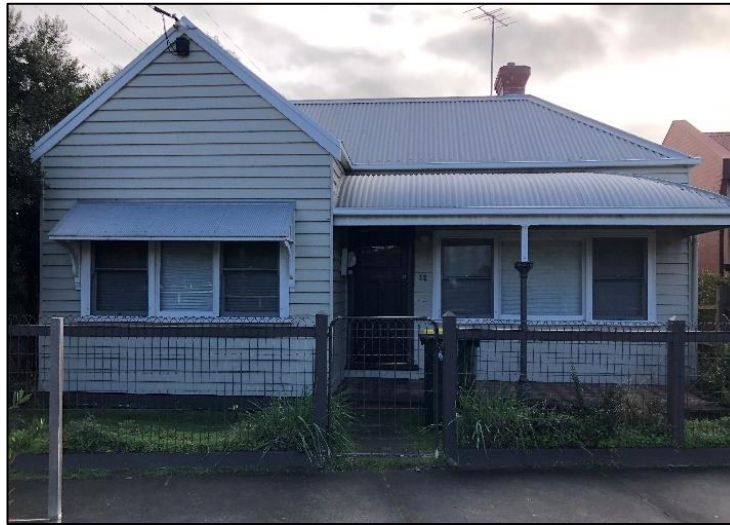
Plate 120: 12 Wharf Street front view
