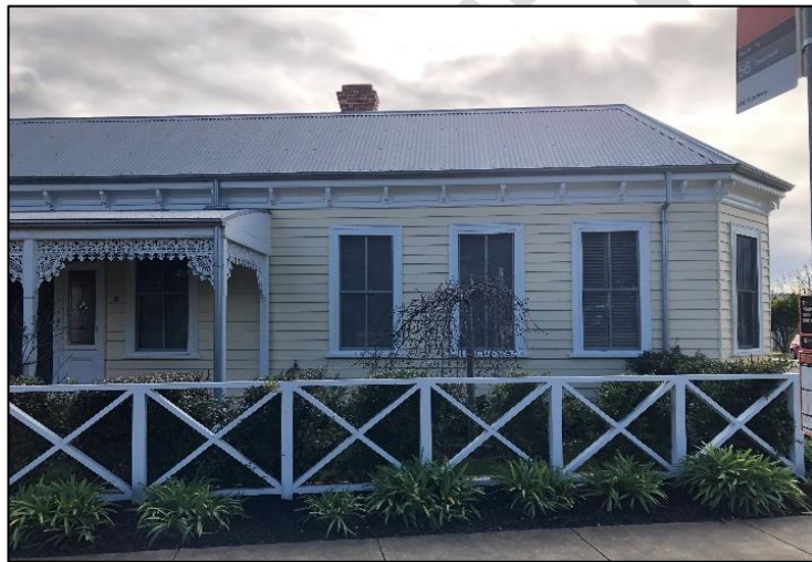
Plate 116: 8 Wharf Street front view
