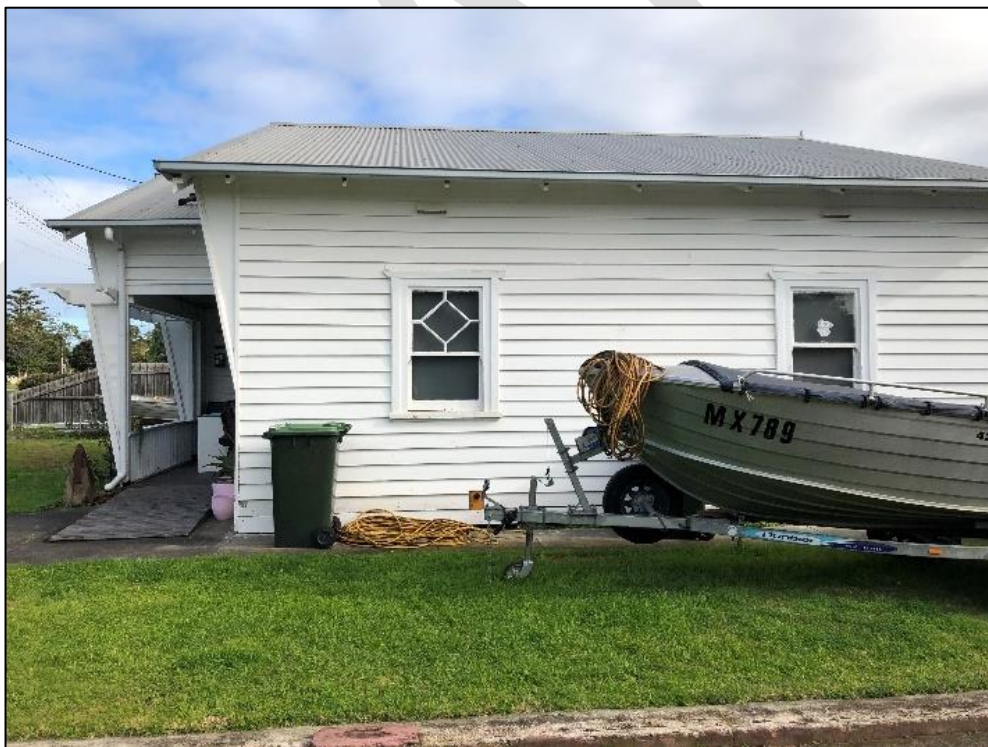
Plate 124: 14 Wharf Street side view
