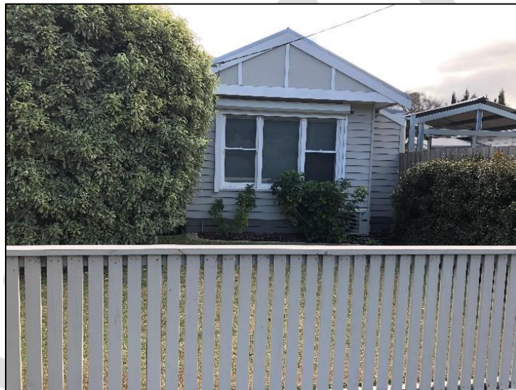
Plate 126: 16 Wharf Street front view
