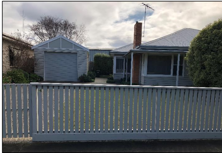
Plate 125: 16 Wharf Street front view
