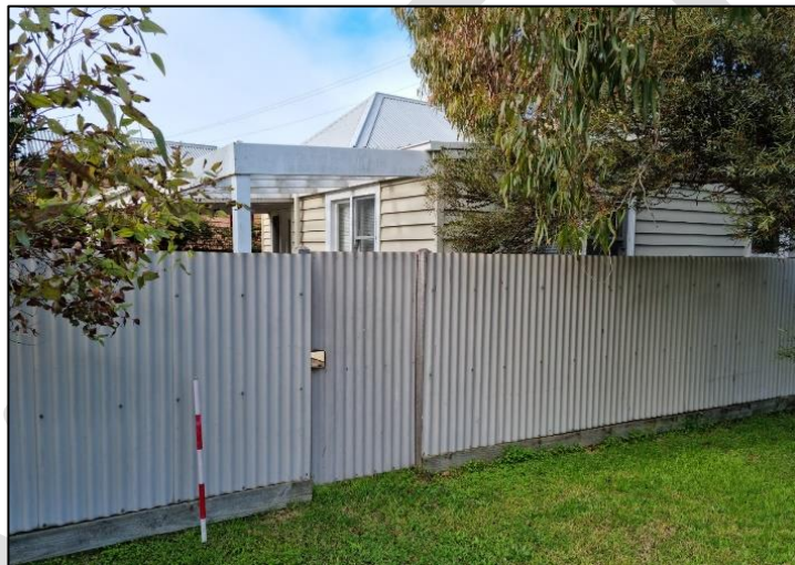
Plate 121: 12 Wharf Street rear view
