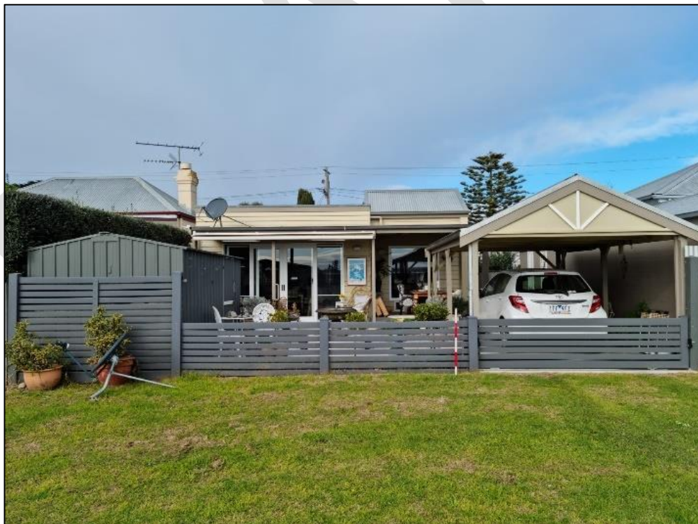
Plate 146: 36 Wharf Street rear view
