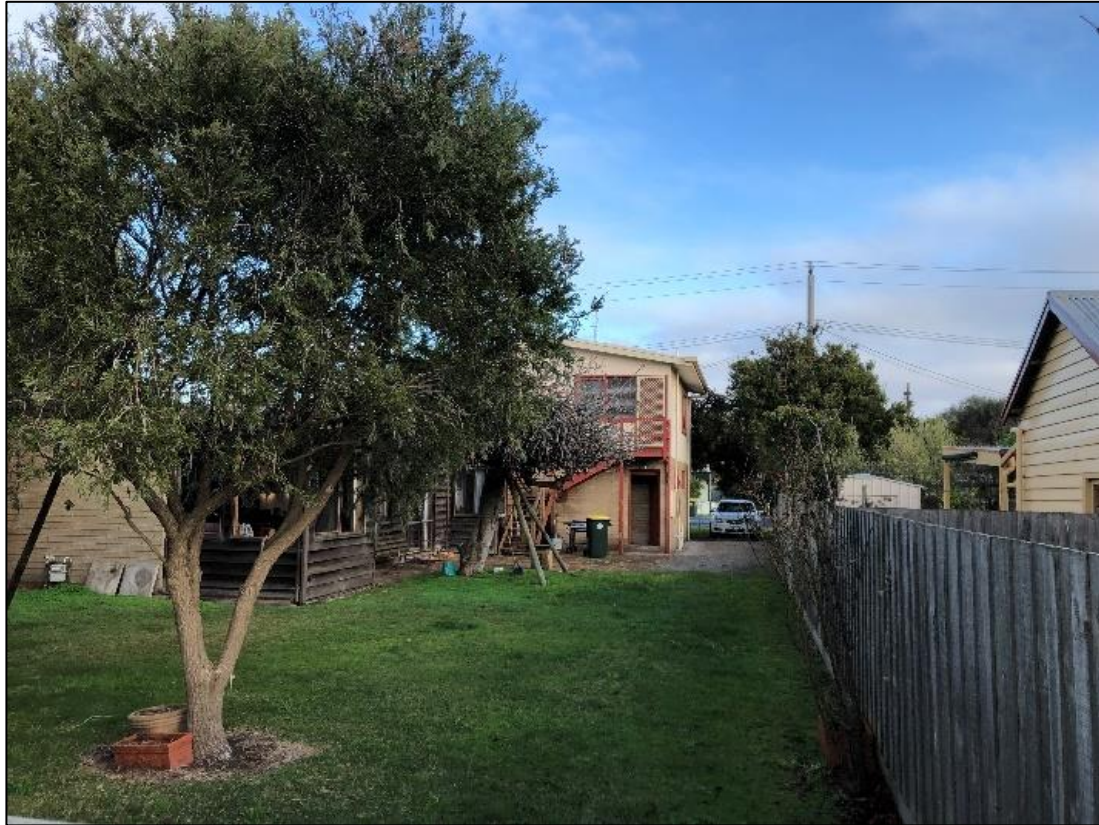
Plate 15: 18 Bay Street front view
