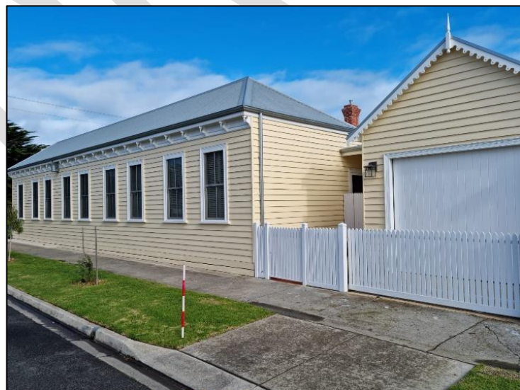
Plate 117: 8 Wharf Street side view
