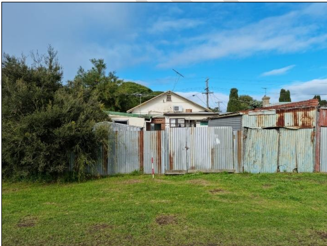
Plate 138: 28 Wharf Street rear view
