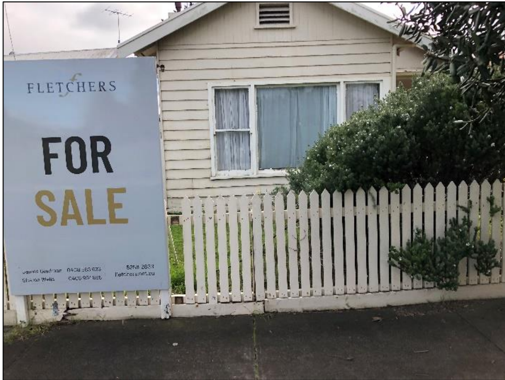
Plate 154: 44 Wharf Street front view
