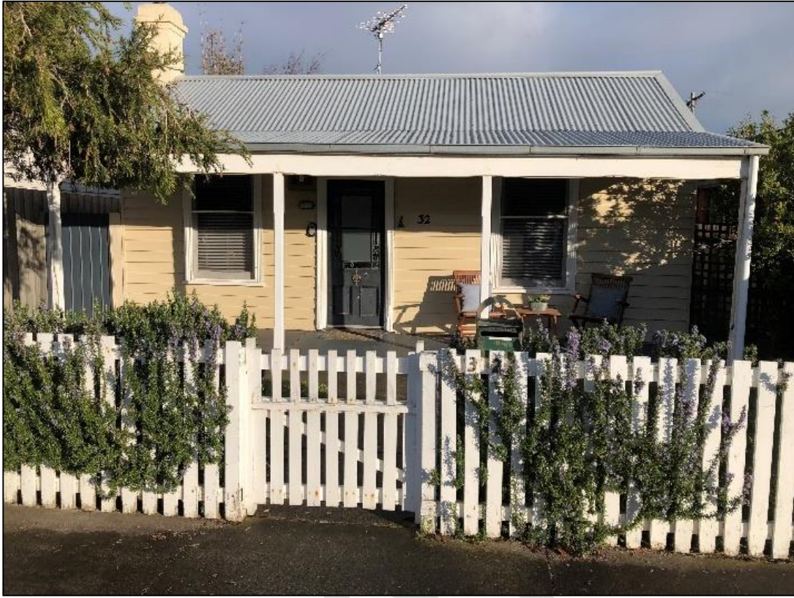
Plate 71: 32 Beach Street front view
