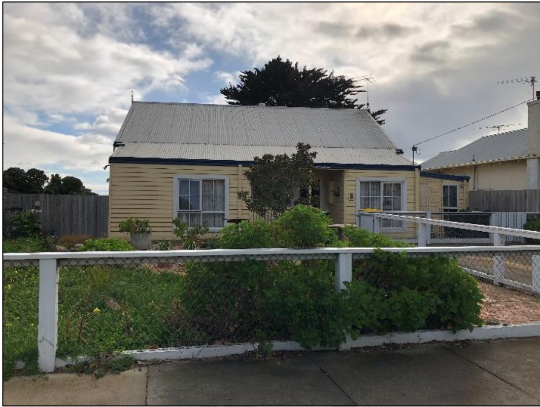
Plate 156: 46 Wharf Street front view
