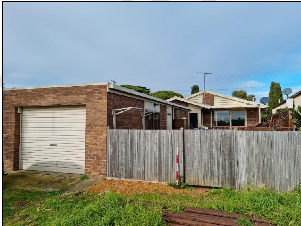
Plate 142: 32 Wharf Street rear view
