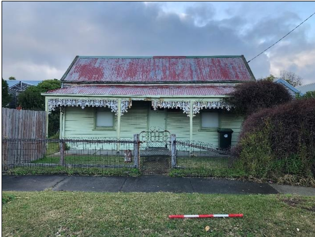
Plate 43: 15 Beach Street front view
