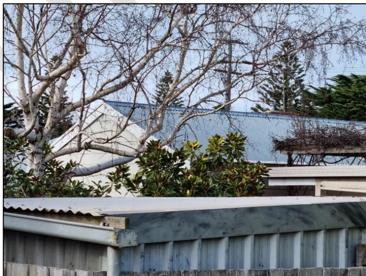
Plate 127: 16 Wharf Street rear view
