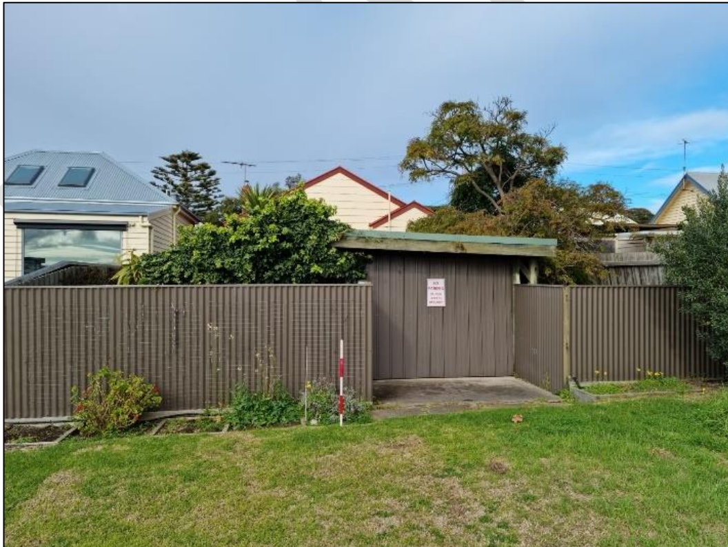
Plate 153: 42 Wharf Street rear view
