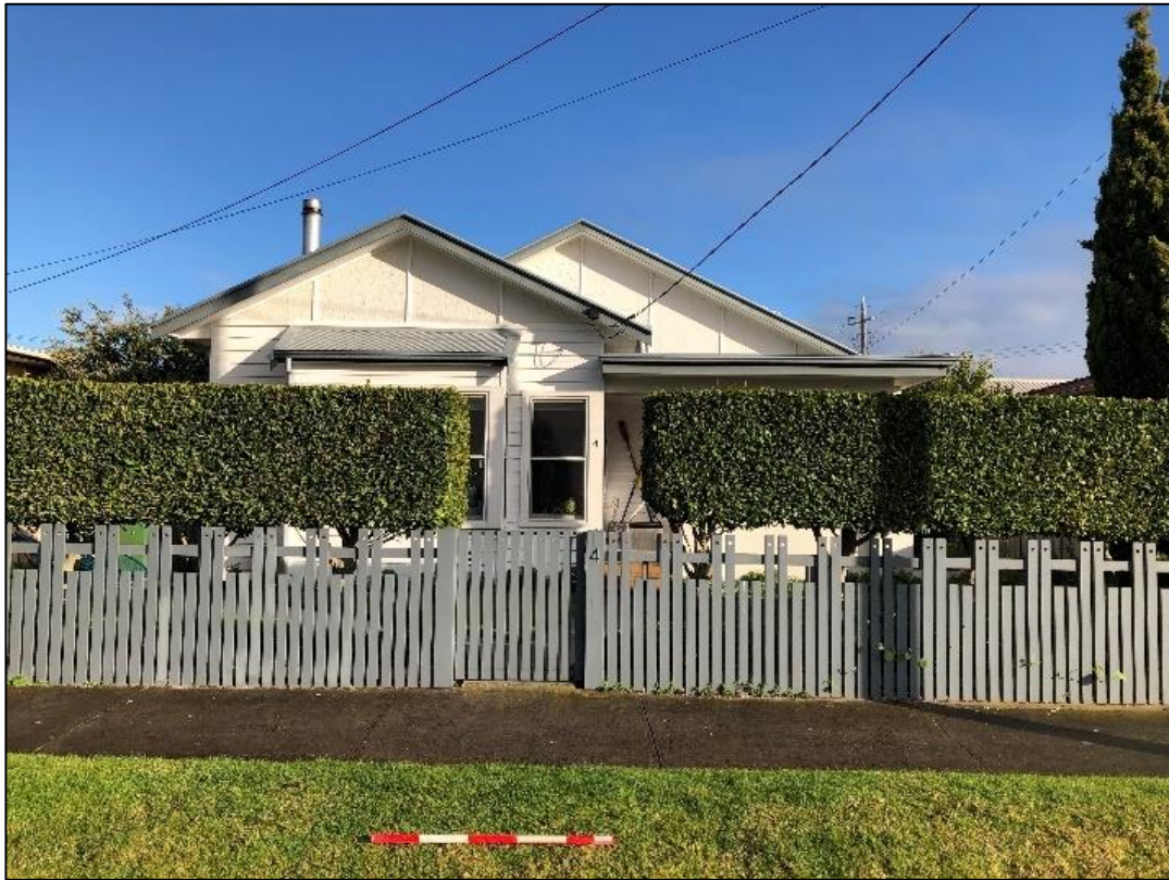
Plate 3: 4 Bay Street front view
