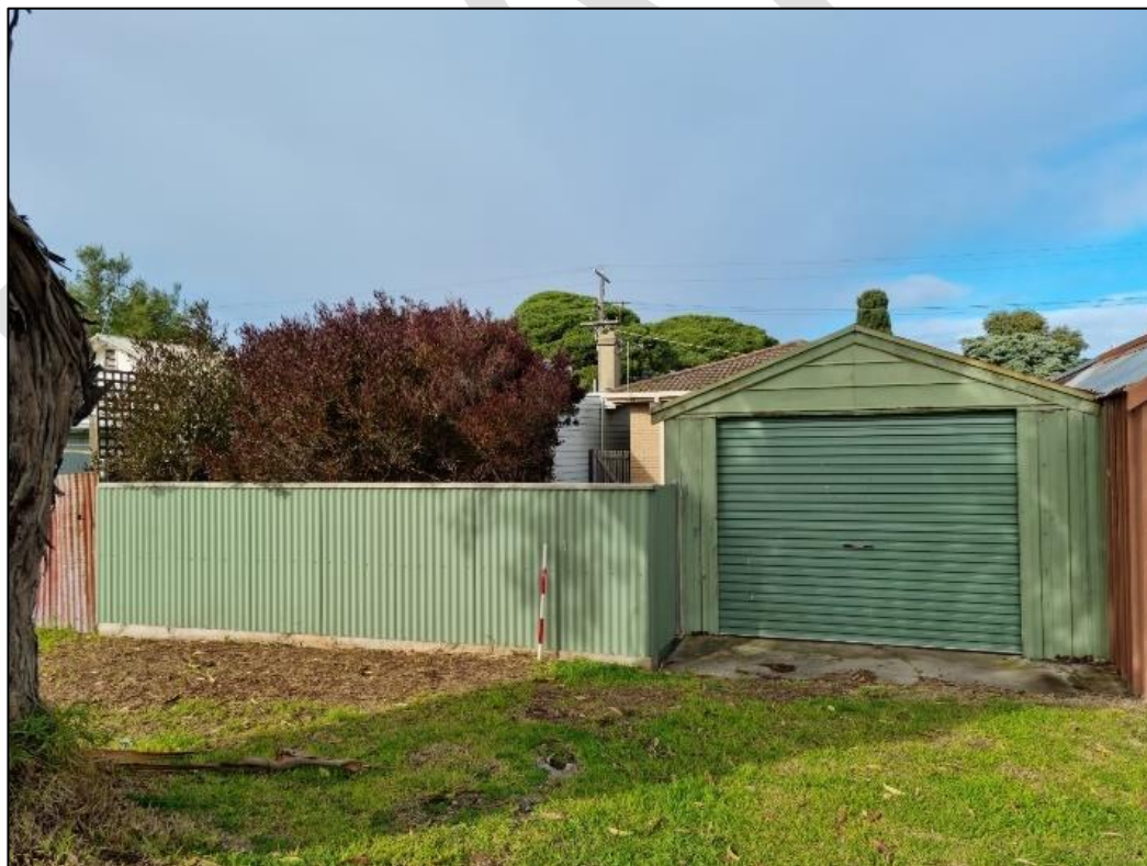
Plate 140: 30 Wharf Street rear view
