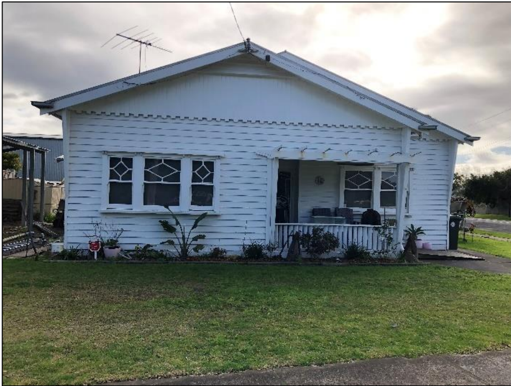
Plate 123: 14 Wharf Street front view
