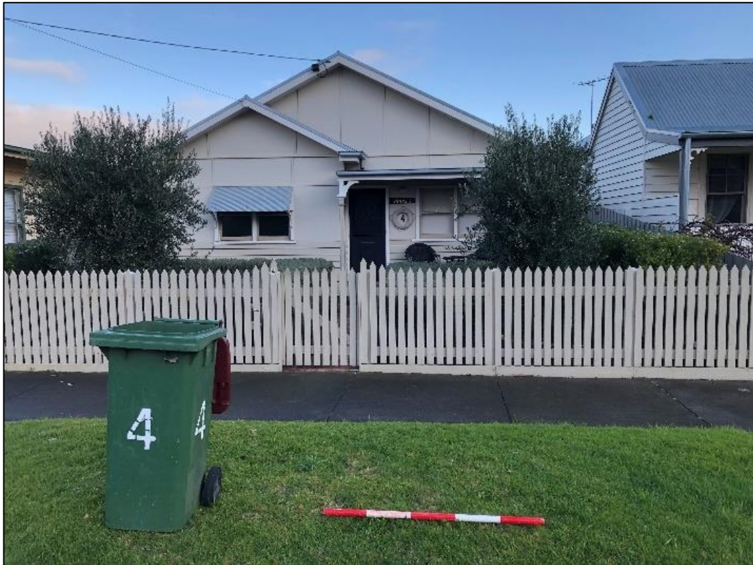
Plate 25: 4 Beach Street front view
