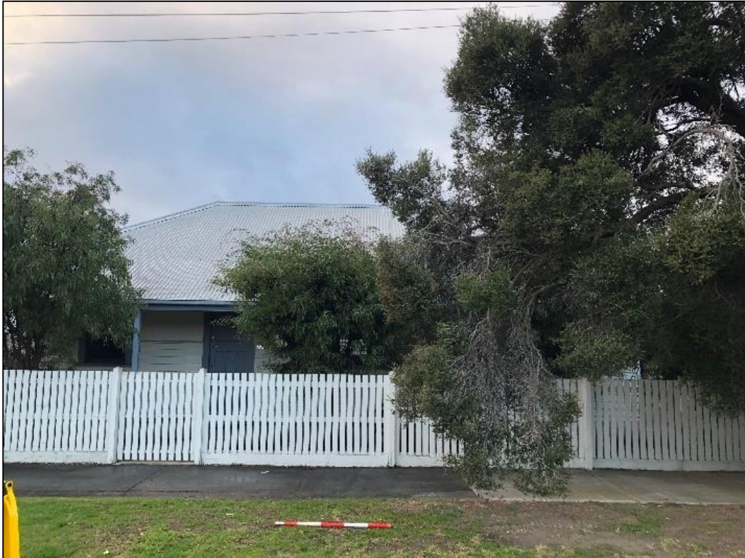
Plate 79: 37 Beach Street front view
