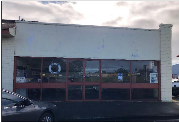
Plate 110: 4 Wharf Street front view
