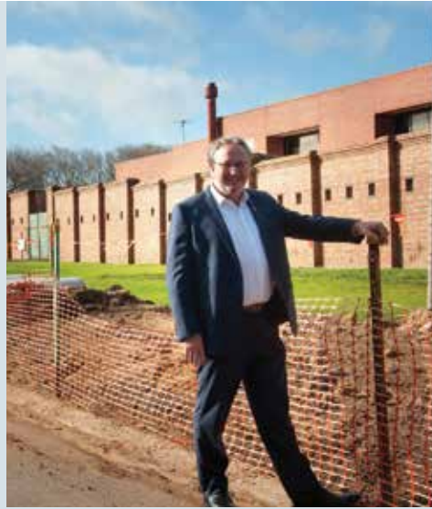
Queenscliffe Mayor Cr Ross Ebbels watched on as construction got underway on Hesse St South in mid-July
