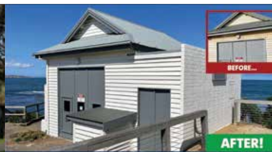
Point Lonsdale's historic 93-year-old foghorn shed has been restored by Council.
