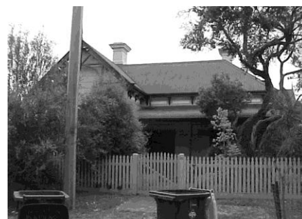
Older single storey buildings
