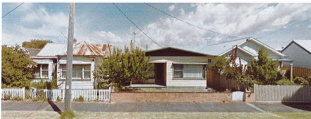
Fig. 2 – Beach Street frontage showing the non-contributory graded house (Google maps)
