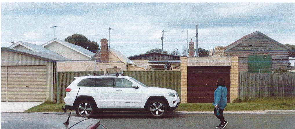
Fig. 5 – Former fisherman’s cottage as viewed from Bay Street
