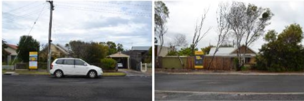
9 Bridge Street as seen from Bridge Street (left) and Harbour Street (right)
