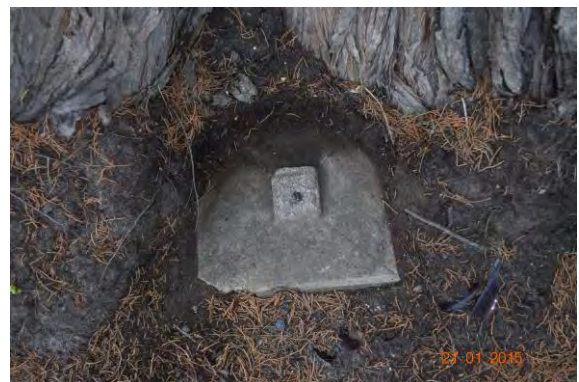
Figure 6: Concrete base at the foot of Tree 12 on Flinders Street suggest that these trees too, were commemorative plantings.
