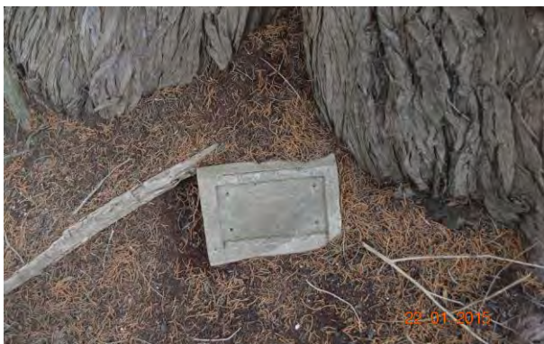
Figure 5: Concrete base at the foot of Tree 25. This tree is one of the 1918 Avenue of Honour trees.
