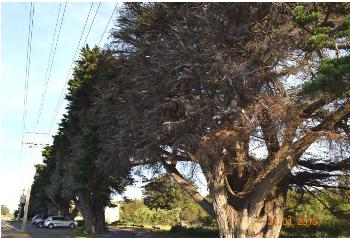
Figure 41: High voltage power line clearance offsets has involved pruning the trees back to bare wood.
