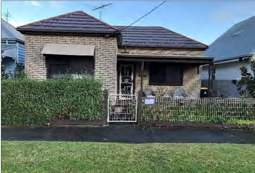
Street frontage of 18 Beach Street
