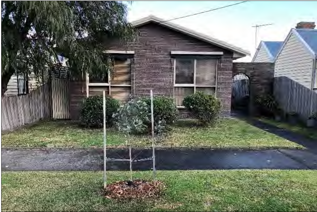
Street frontage of 10 Beach Street
