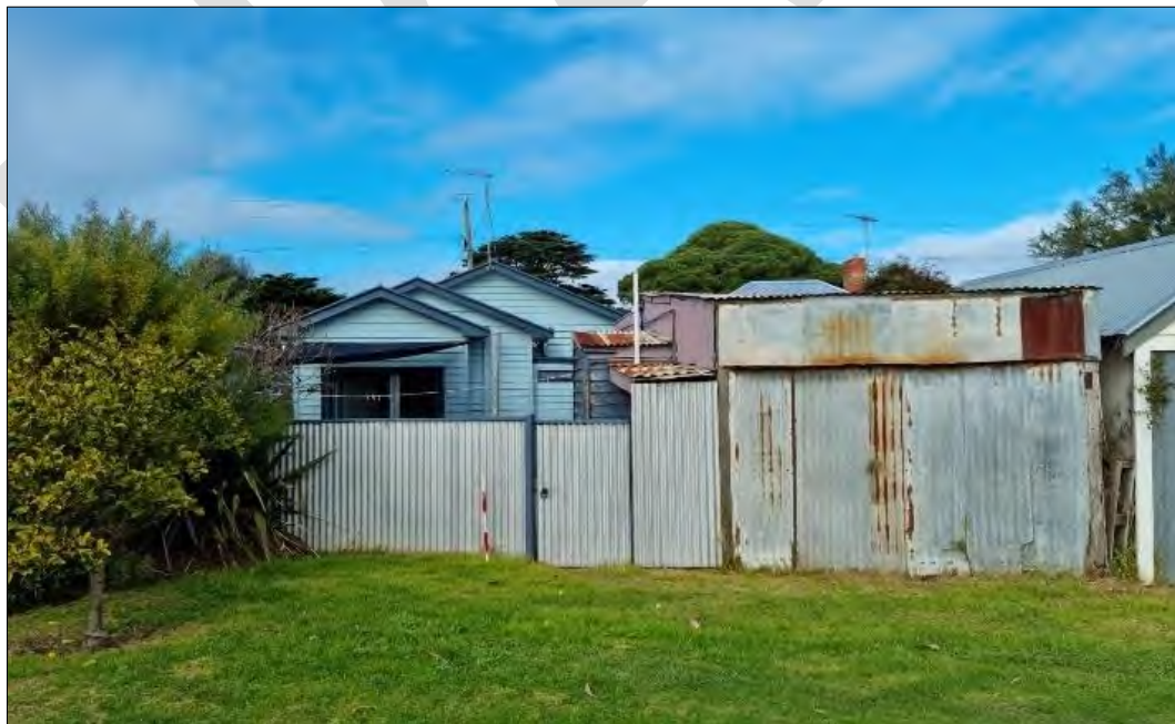
Rear view of 20 Wharf Street
