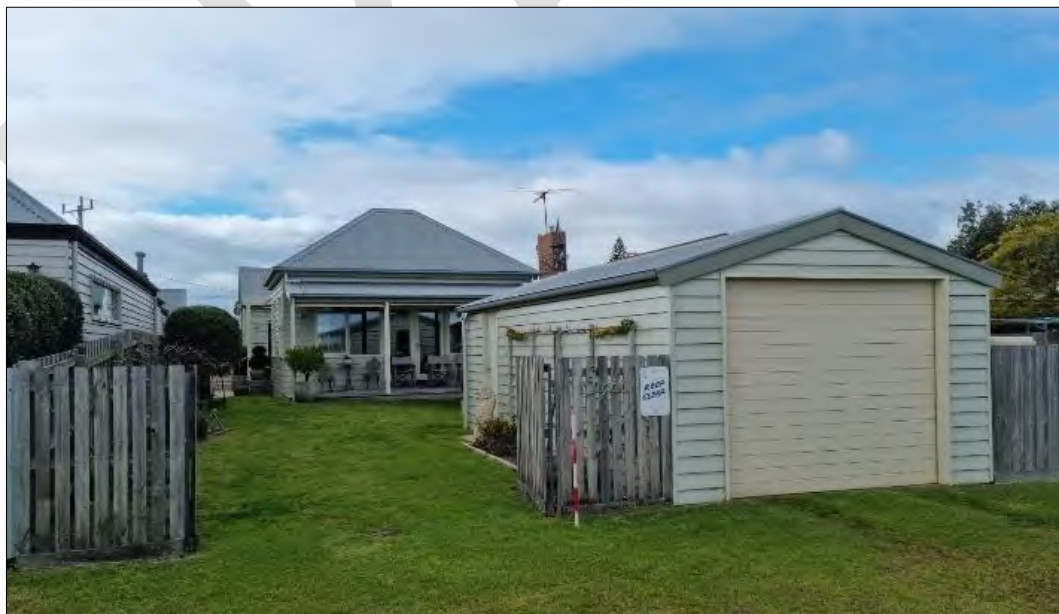
Rear view of 8 Bridge Street
