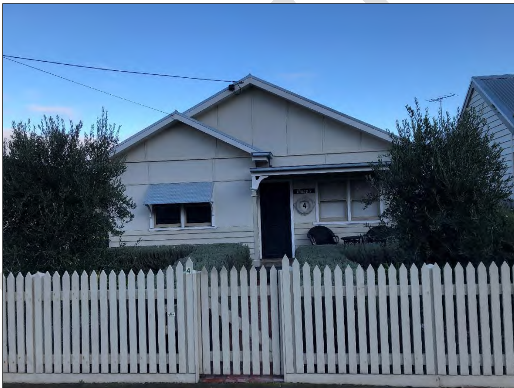
Street frontage of 4 Beach Street
