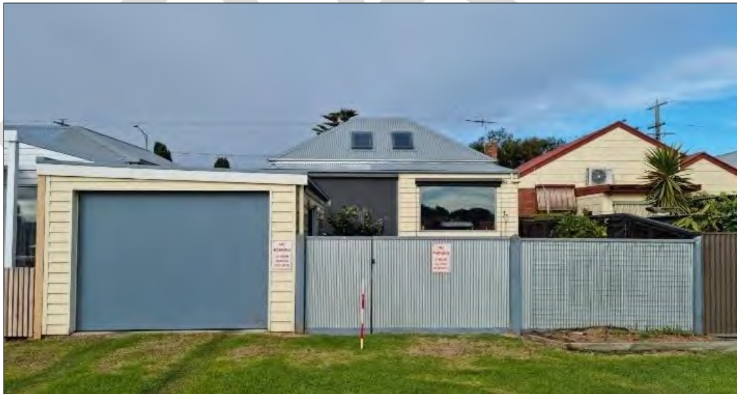
Rear view of 40 Wharf Street
