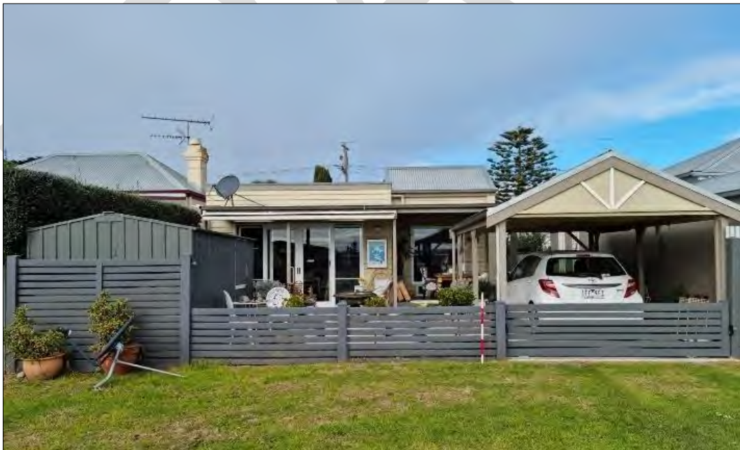
Rear view of 36 Wharf Street
