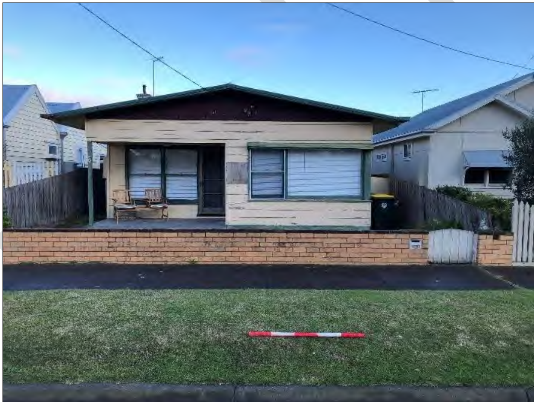
Street frontage of 6 Beach Street
