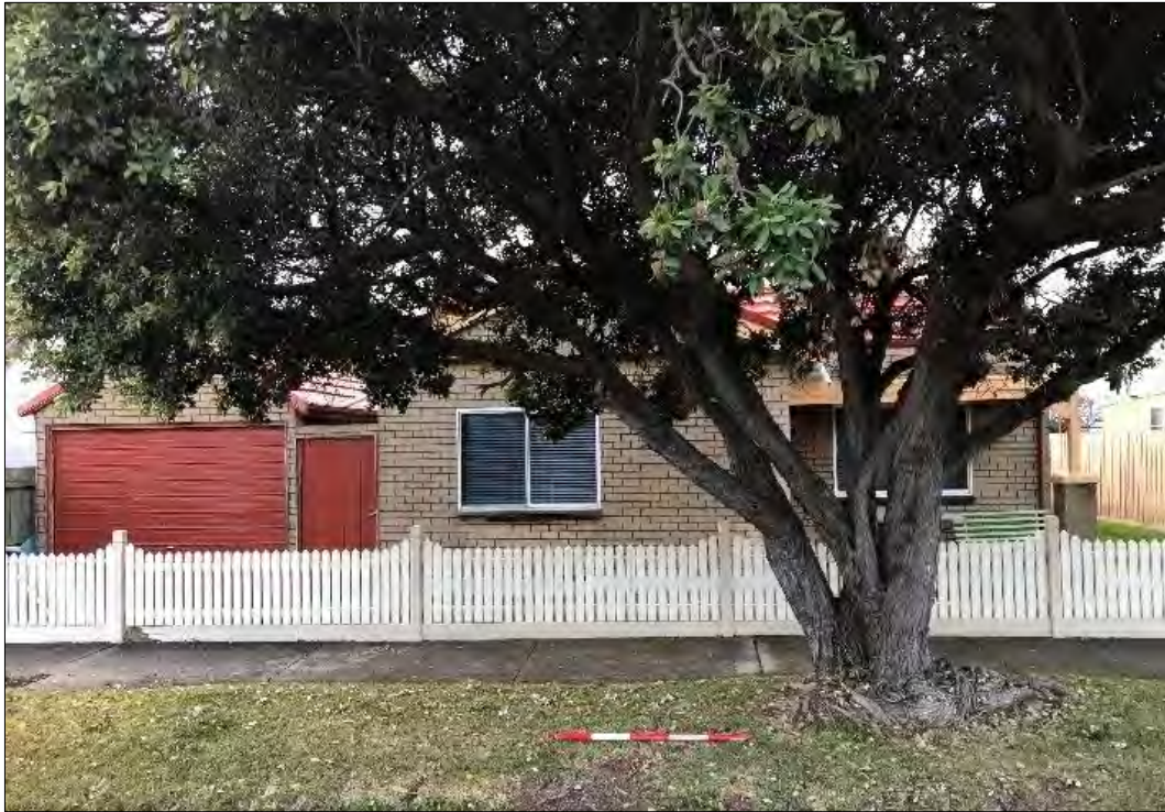
Street frontage of 23 Beach Street
