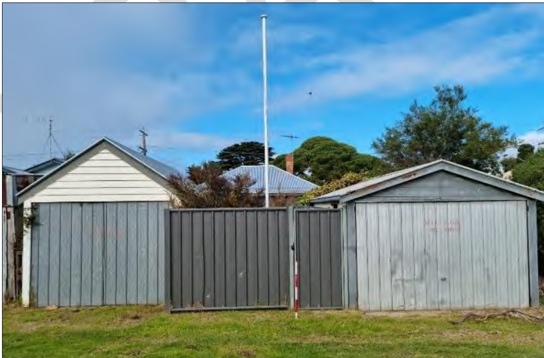
Rear view of 22 Wharf Street
