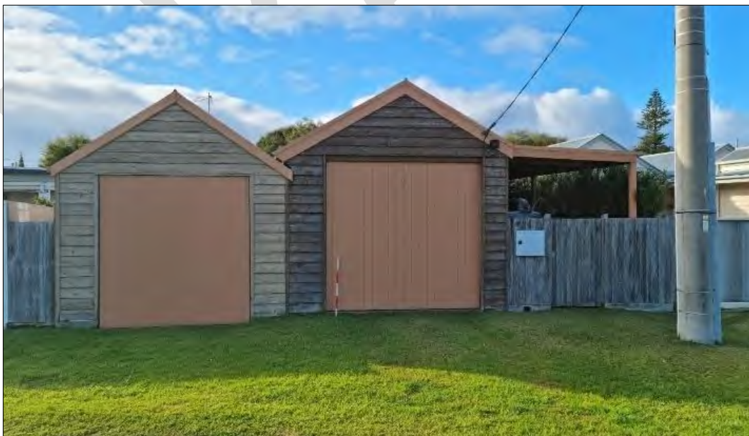
Rear view of 8 Bay Street, weatherboard sleepout on left
