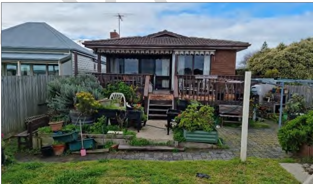
Rear view of 10 Bridge Street
