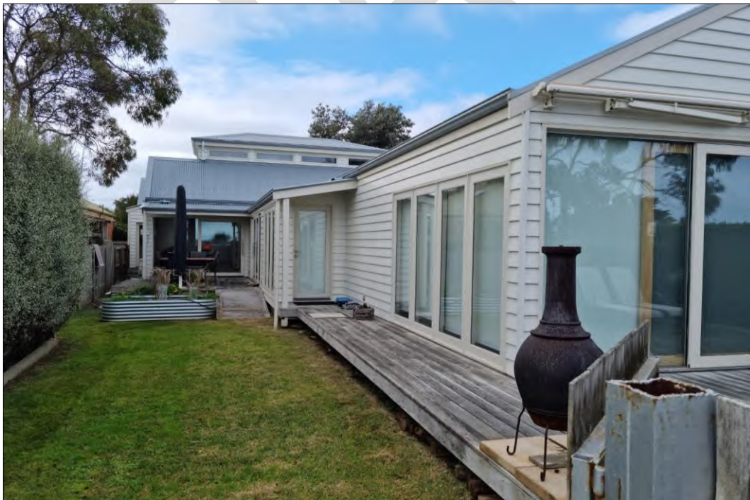
Rear view of 16 Bridge Street
