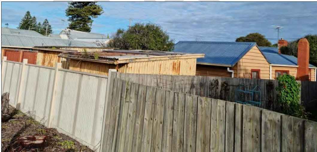
Rear view of 23 Beach Street, noting secondary cottages on right (brick chimney) and left (double wooden doors)
