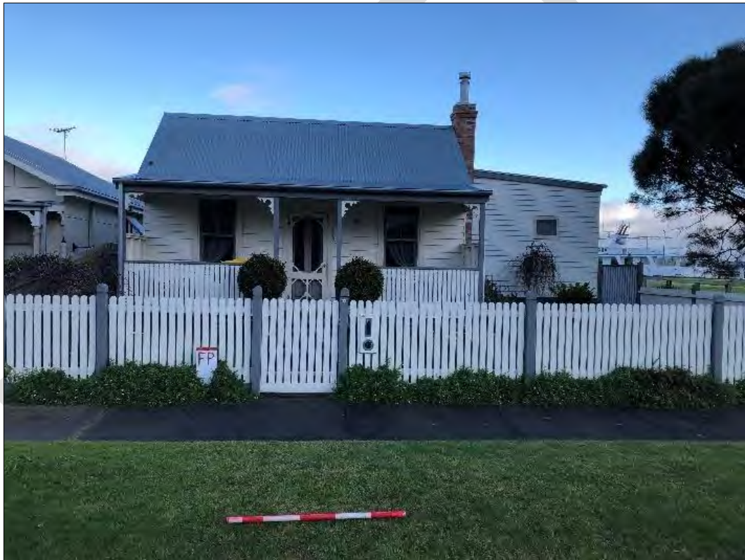
Street frontage of 2 Beach Street
