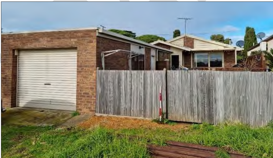
Rear view of 32 Wharf Street
