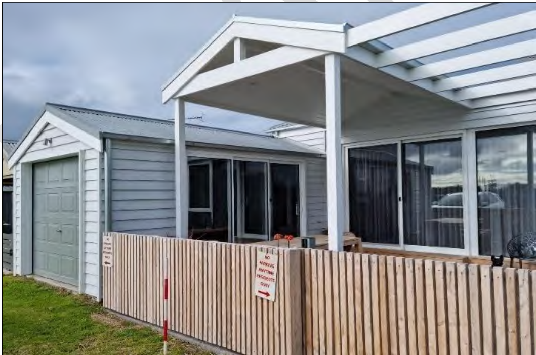
Rear view of 38 Wharf Street
