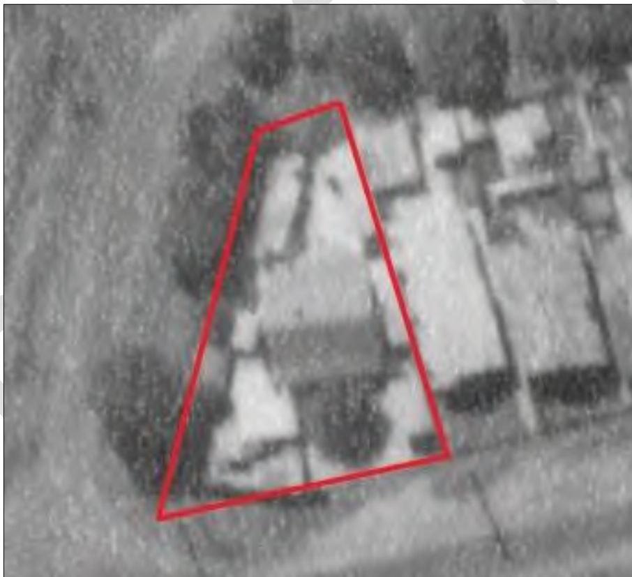
Aerial photograph of 46 Wharf Street dated 1957 (Source: LANDATA 2023).
