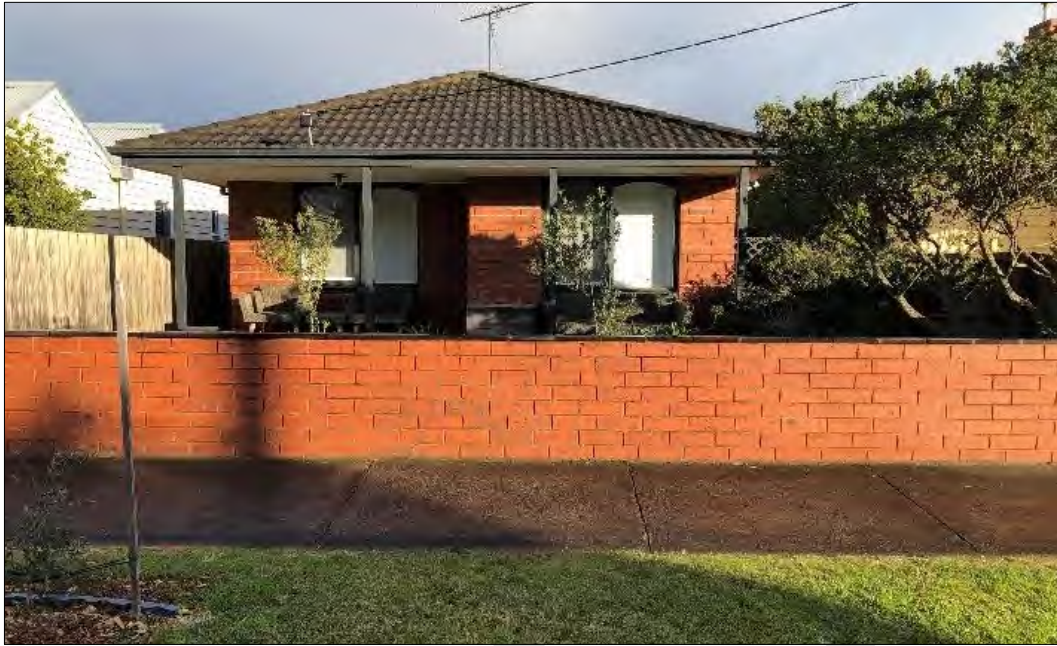
Street frontage of 30 Beach Street
