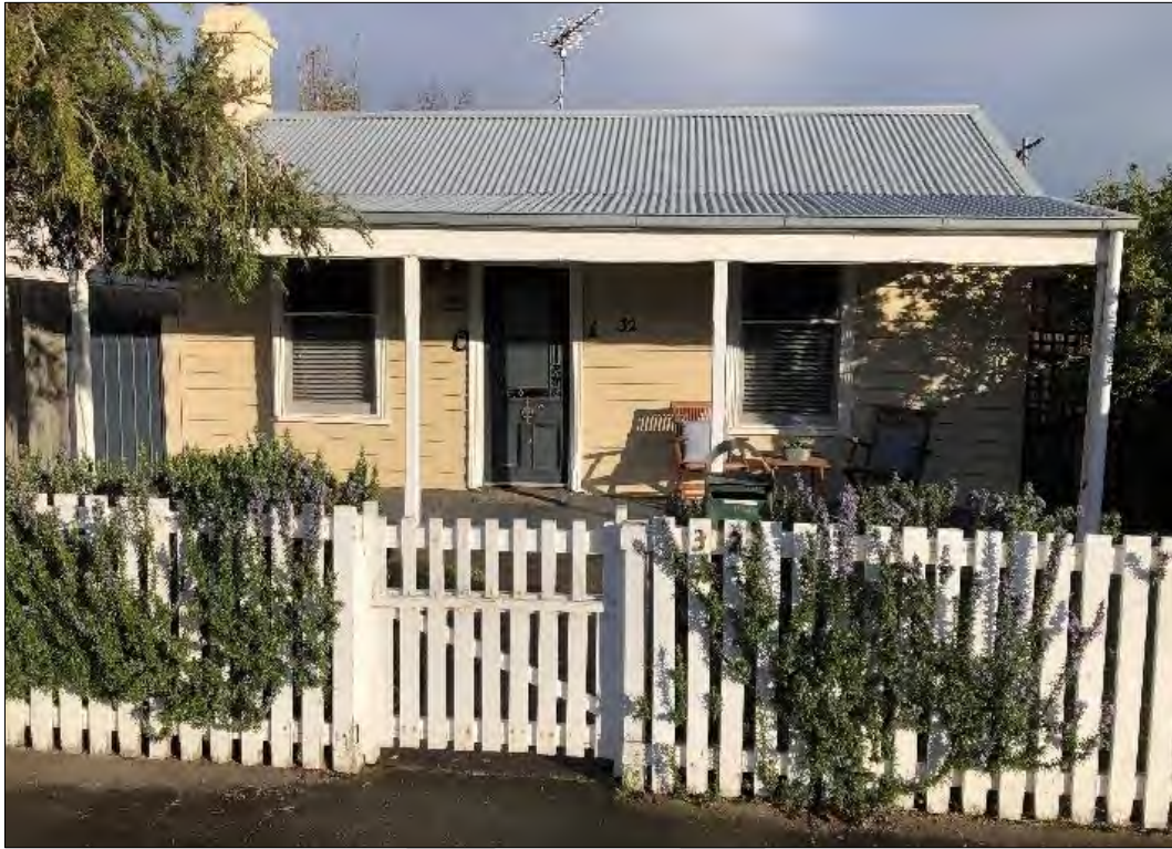
Street frontage of 32 Beach Street
