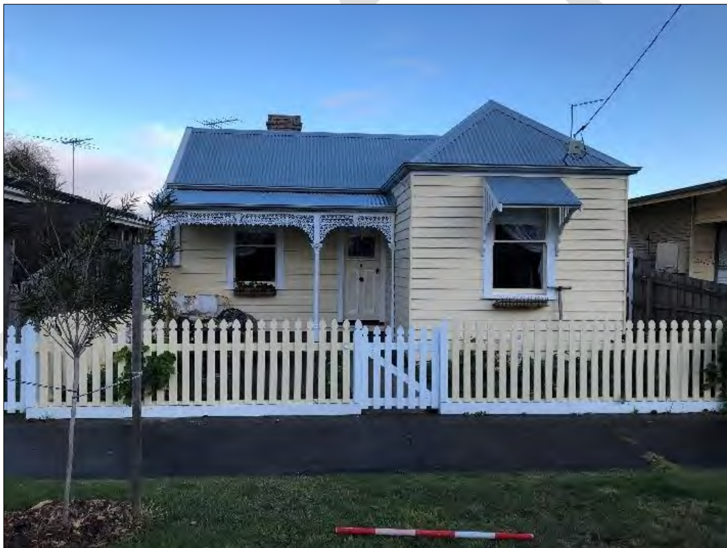
Street frontage of 8 Beach Street
