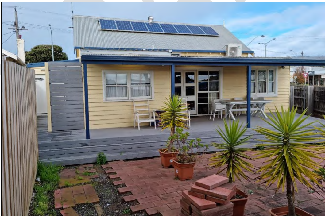
Rear view of 46 Wharf Street
