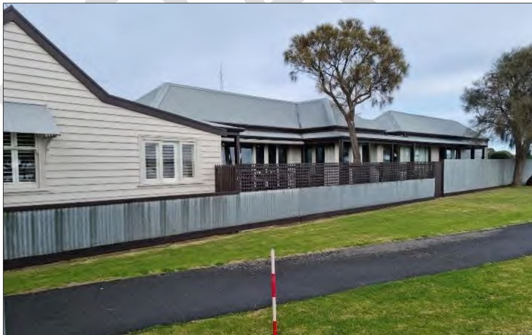
North-facing view of 6 Bridge Street
