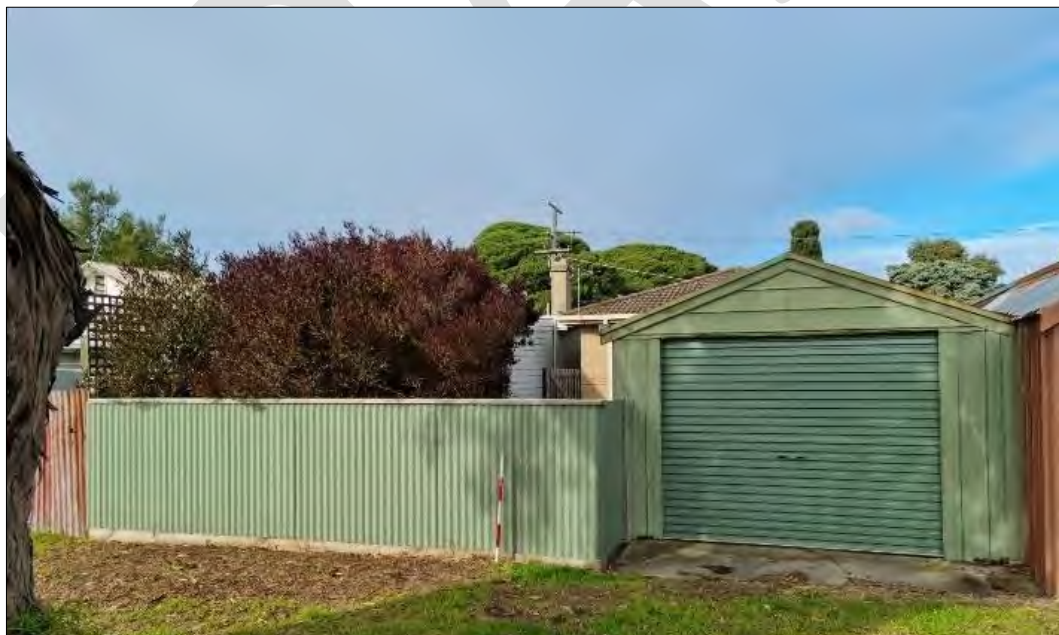
Rear view of 30 Wharf Street
