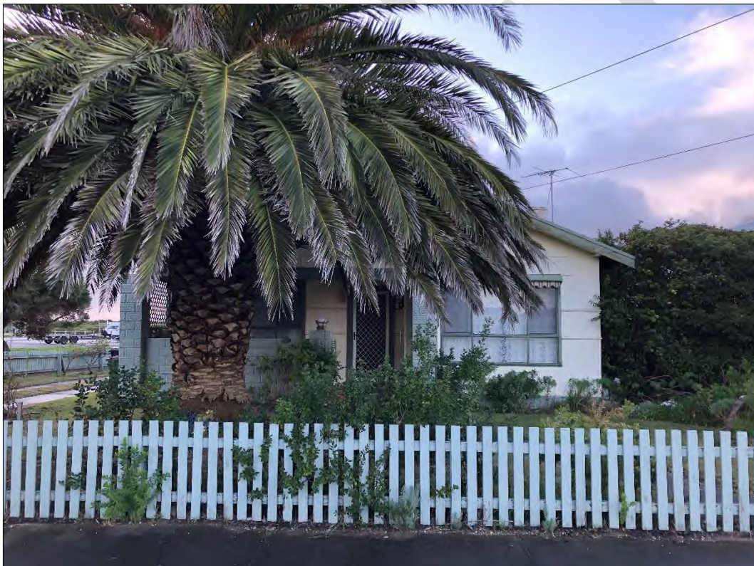
Street frontage of 5 Beach Street
