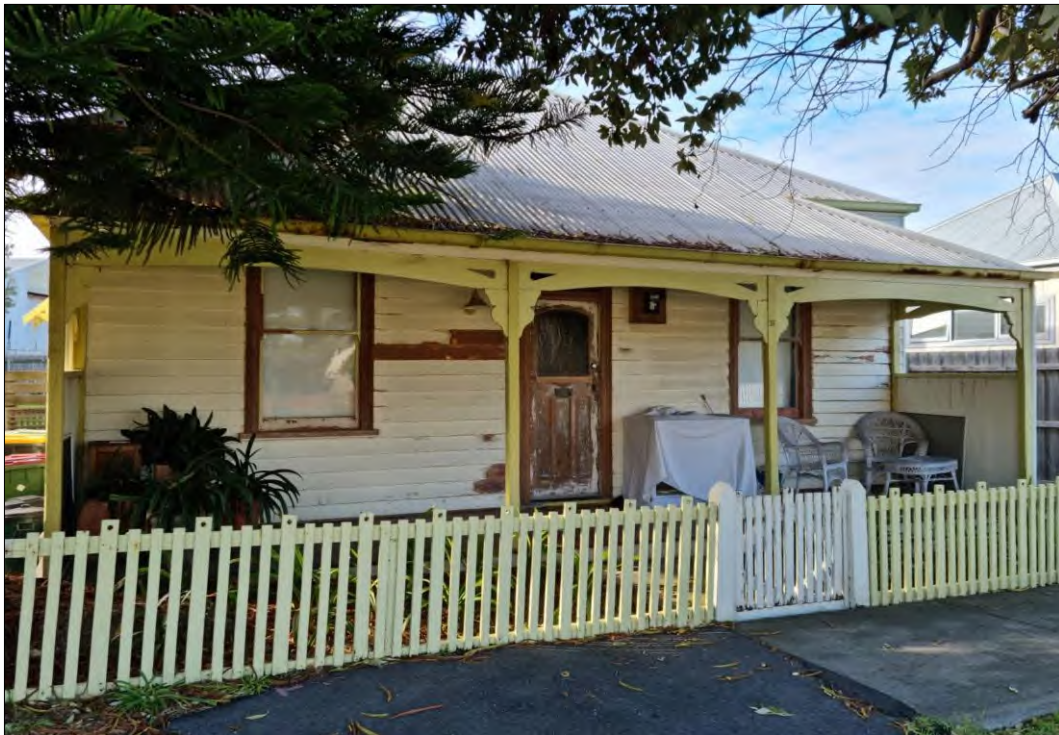
Street frontage of 35 Beach Street
