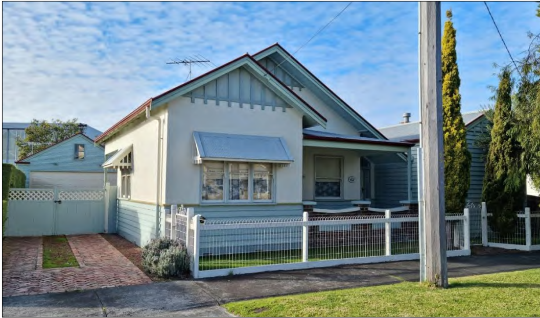
Street frontage of 31 Beach Street, note sleepout alongside dwelling (right)
