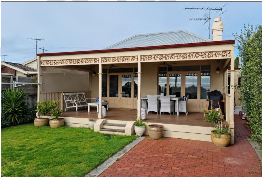
Rear view of 34 Wharf Street
