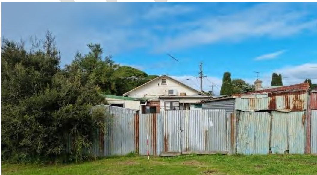
Rear view of 26 Wharf Street
