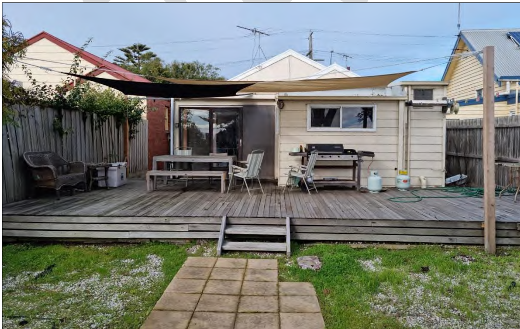
Rear view of 44 Wharf Street
