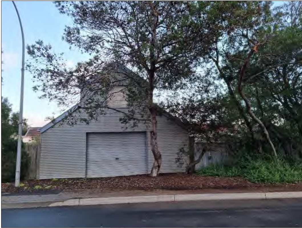
Two-storey garage facing Harbour Street
