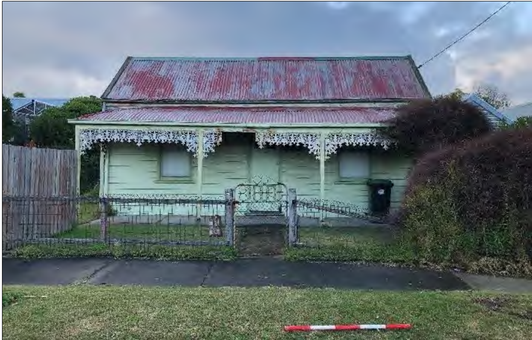
Street frontage of 15 Beach Street
