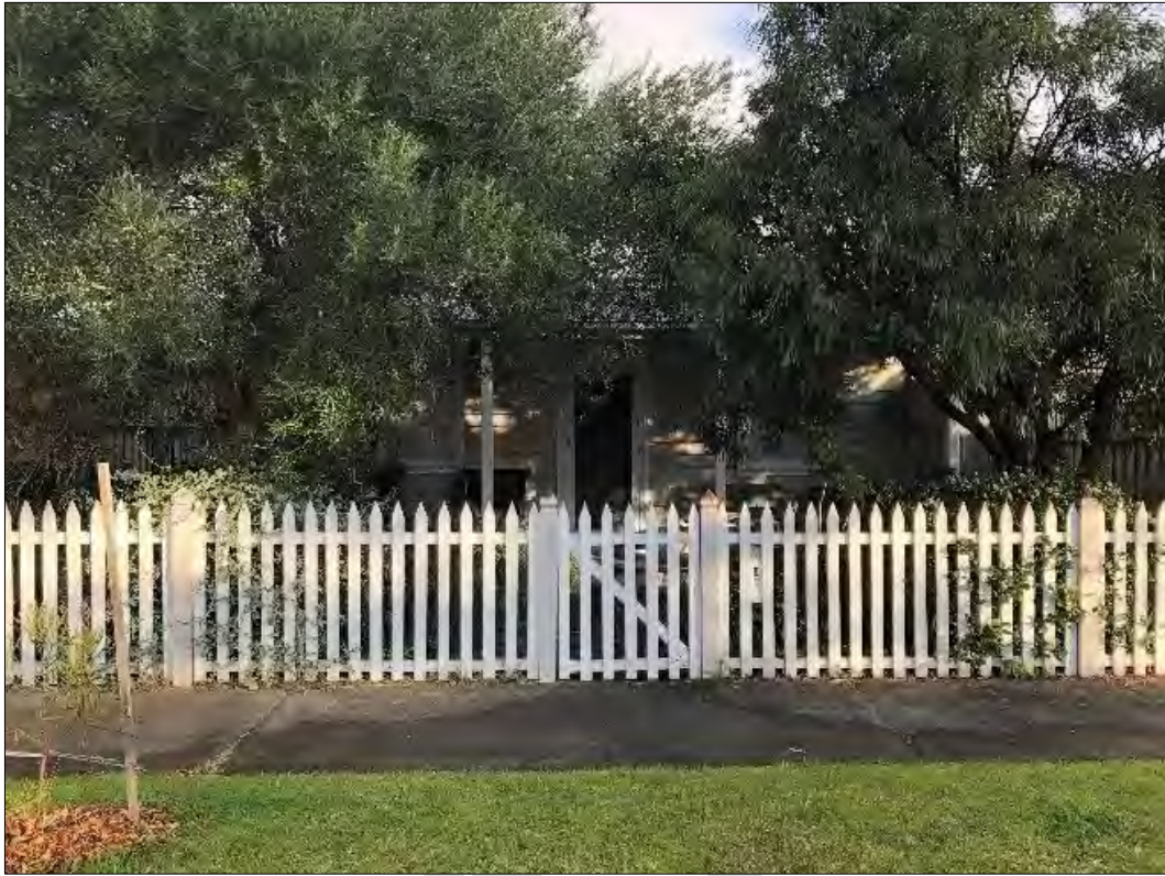
Street frontage of 34 Beach Street
