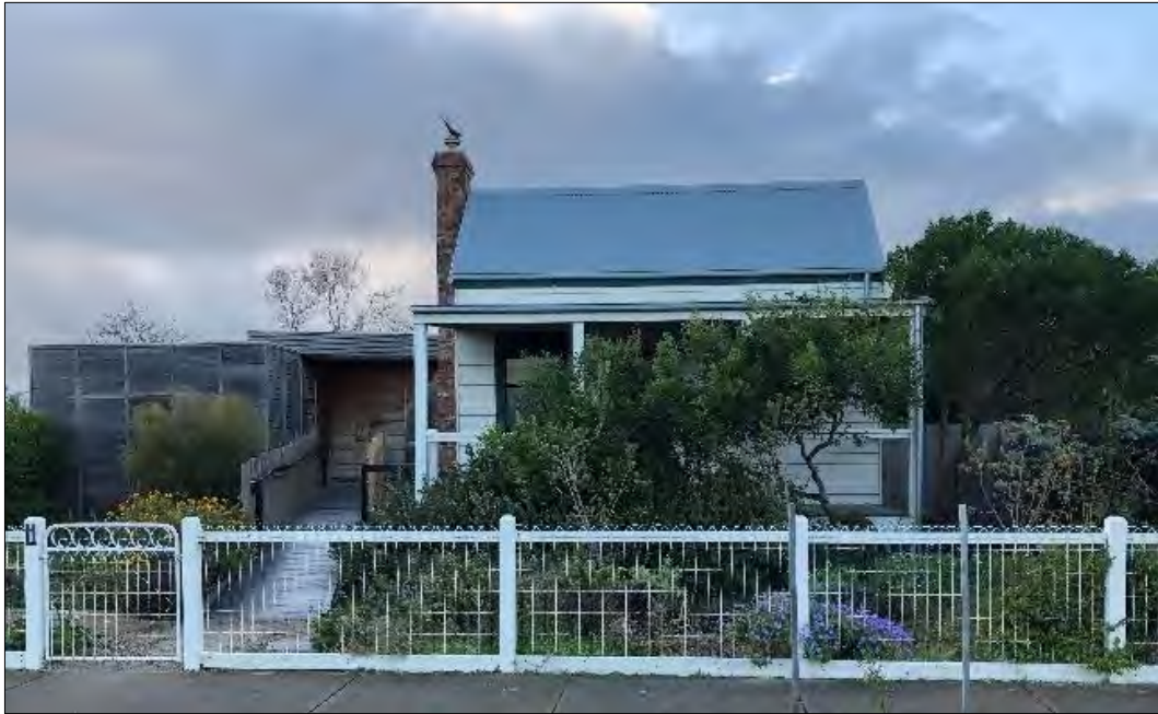
Street frontage of 11 Beach Street
