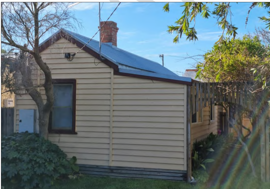
Weatherboard sleepout in rear of 16 Bay Street
