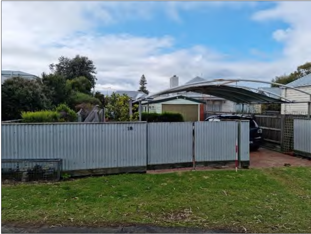
Rear view of 18 Bridge Street
