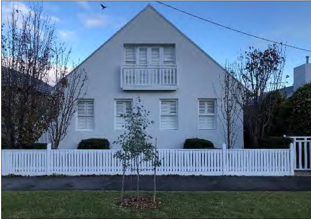
Street frontage of 16 Beach Street
