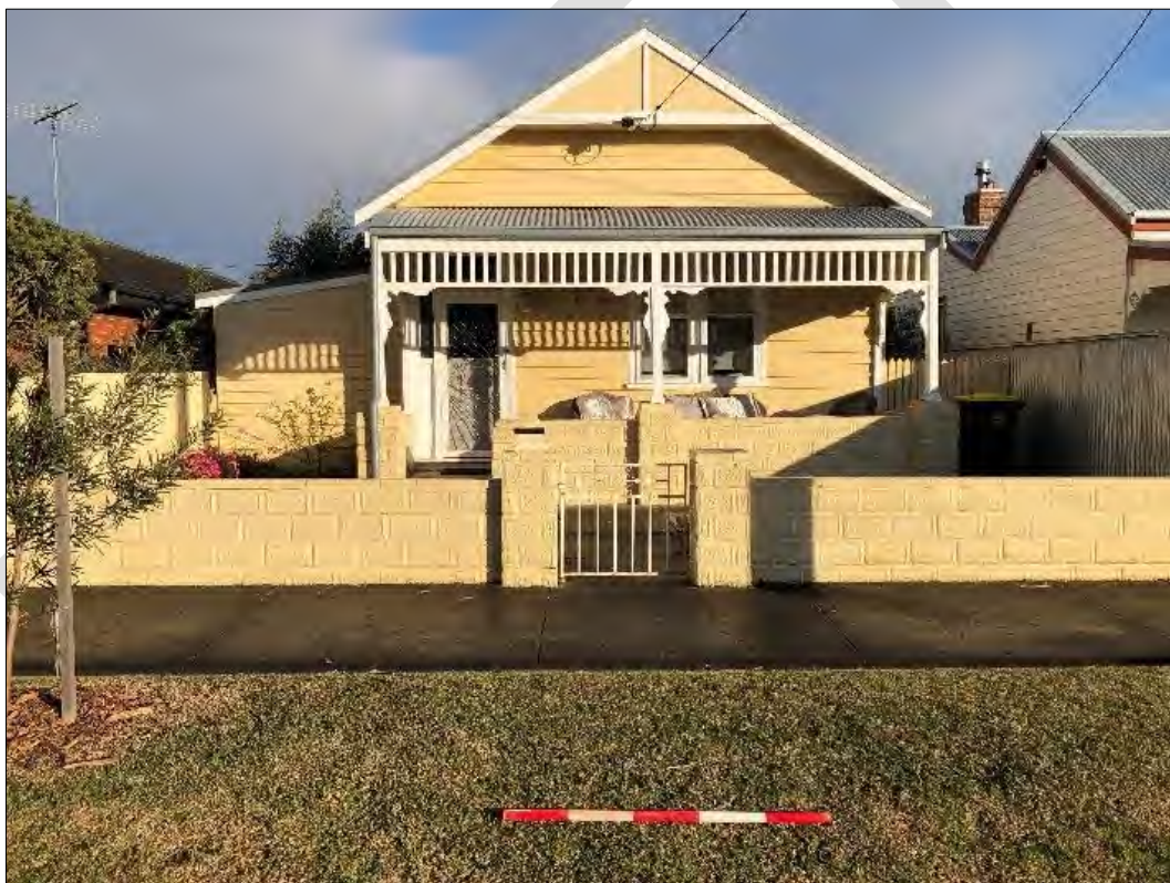
Street frontage of 28 Beach Street
