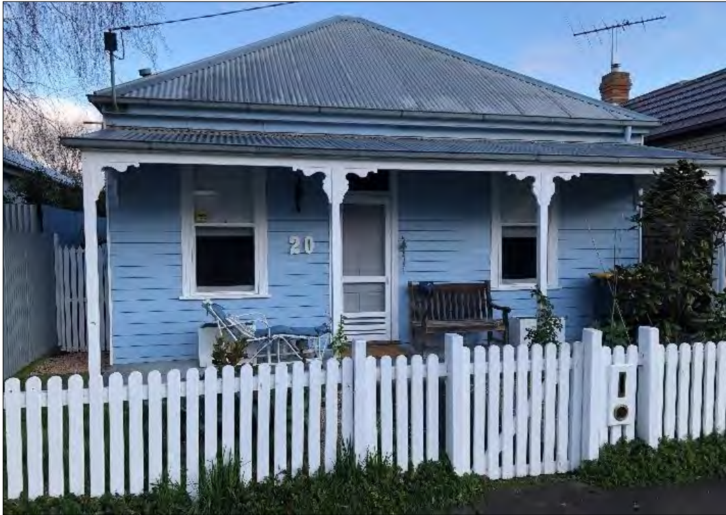
Street frontage of 20 Beach Street
