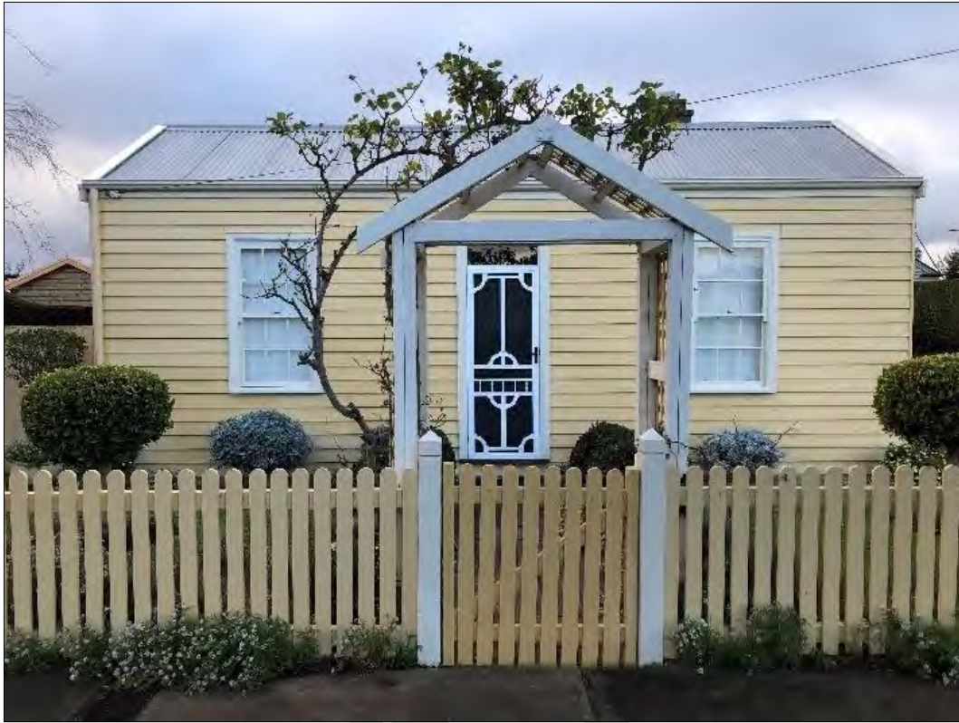
Street frontage of 27 Beach Street
