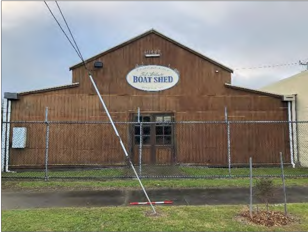
Street frontage of 39 Beach Street
