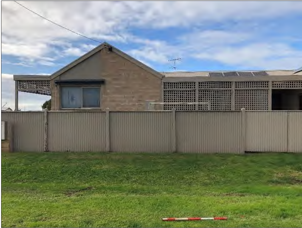
West-facing view of 1 Bridge Street
