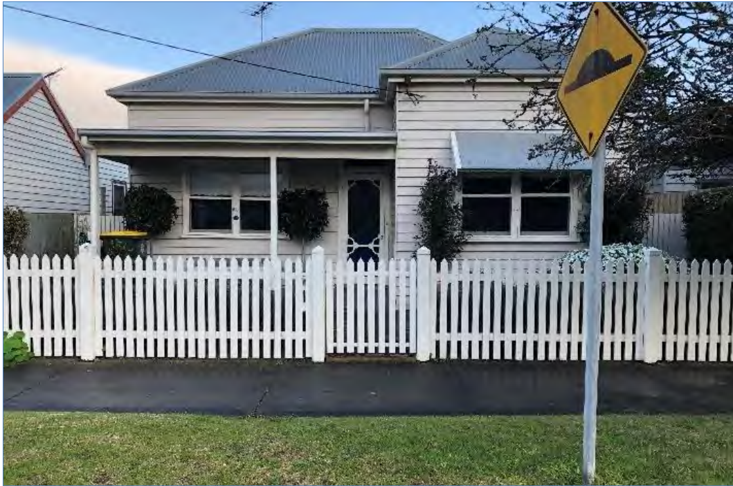
Street frontage of 24 Beach Street
