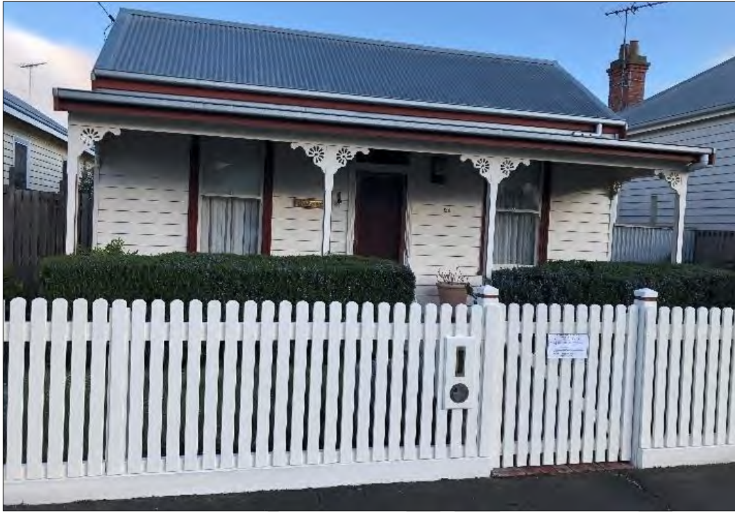
Street frontage of 26 Beach Street
