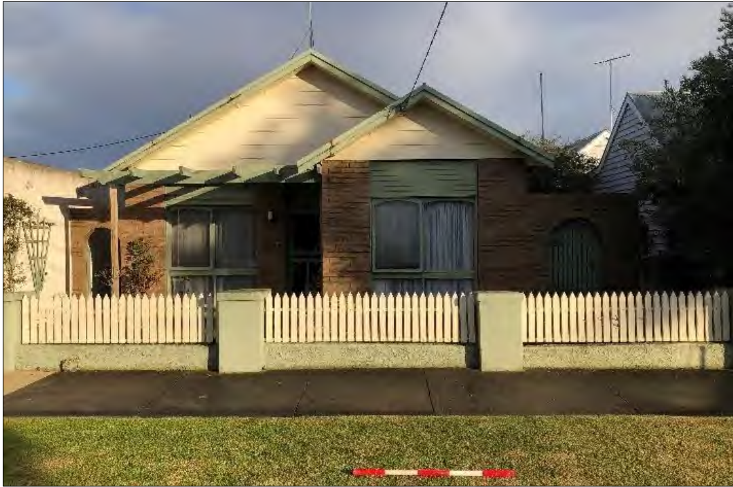
Street frontage of 36 Beach Street
