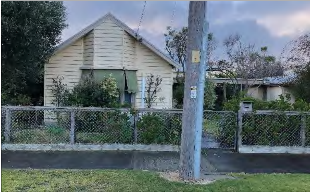
Street frontage of 9 Beach Street
