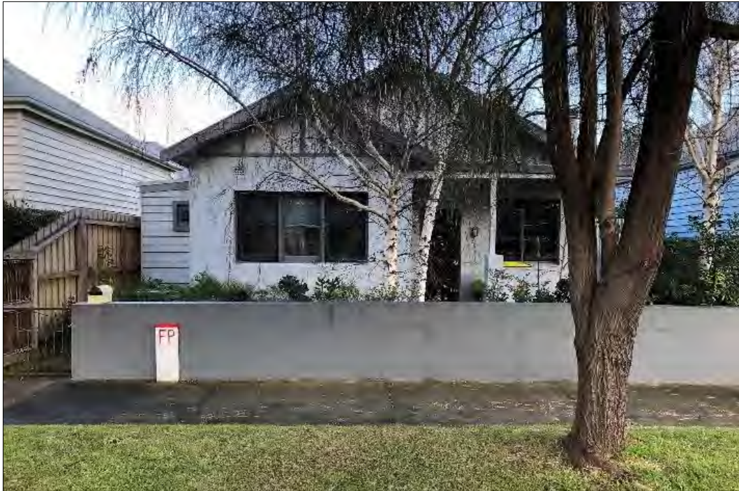
Street frontage of 22 Beach Street
