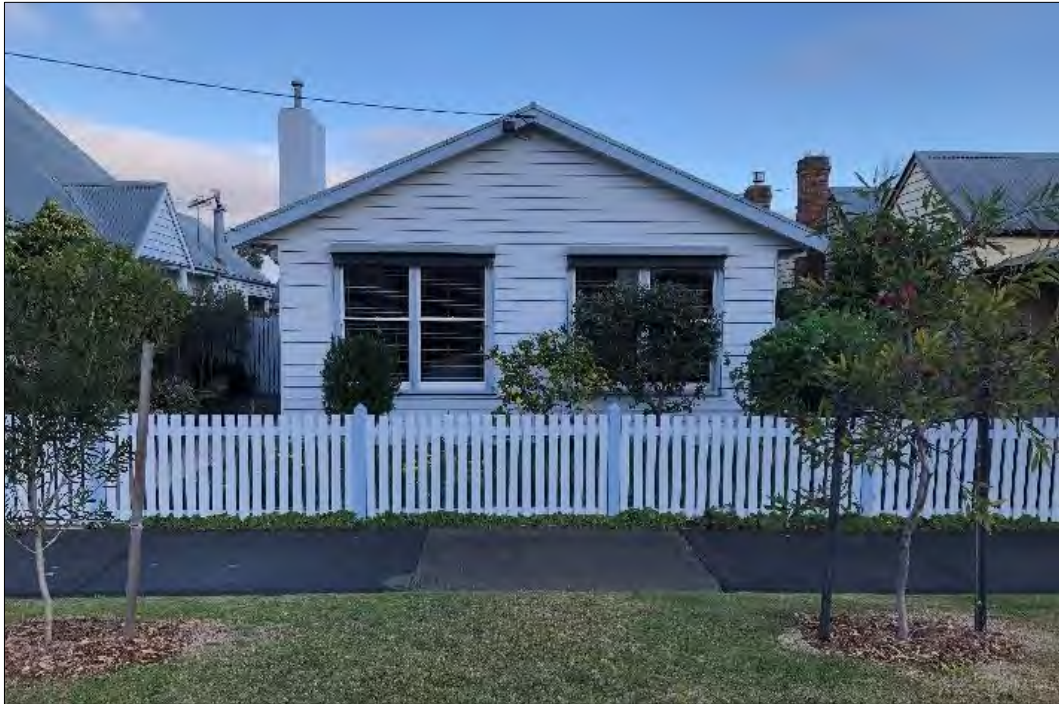
Street frontage of 14 Beach Street
