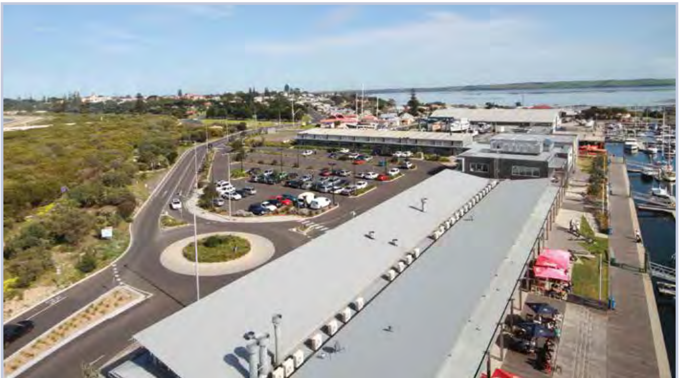
The Ferry to Pier path links the Queenscliff ferry terminal and the Queenscliff pier.
