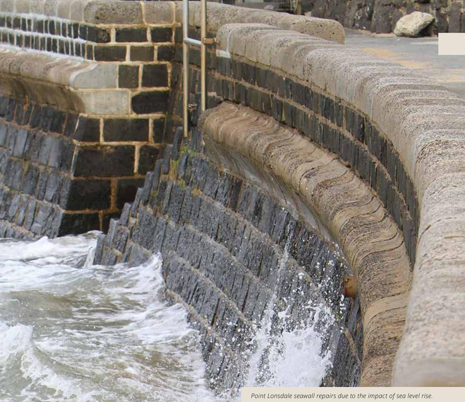
*Point Lonsdale seawall repairs due to the impact of sea level rise.*
