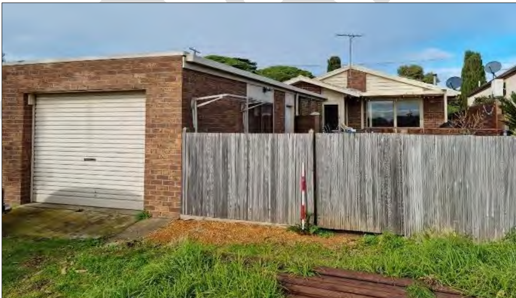
Rear view of 32 Wharf Street
