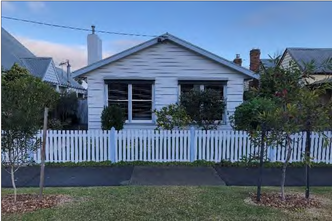
Street frontage of 14 Beach Street
