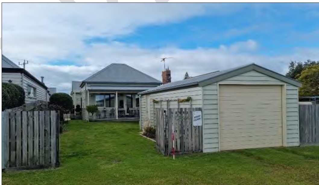
Rear view of 8 Bridge Street
