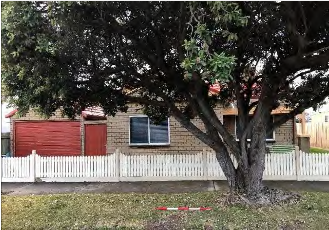
Street frontage of 23 Beach Street
