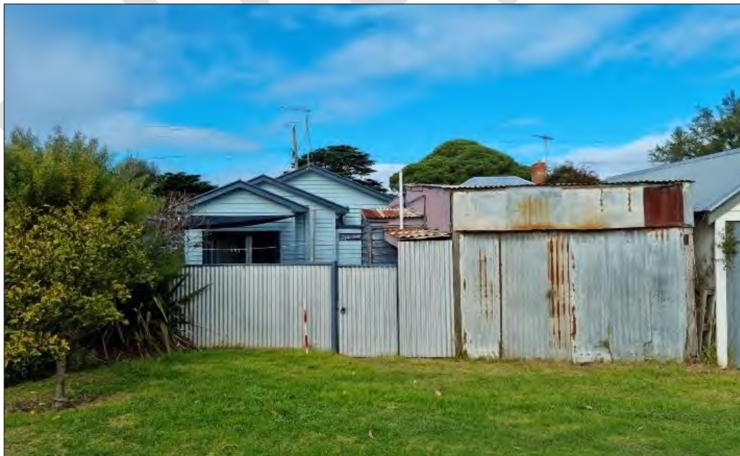
Rear view of 20 Wharf Street
