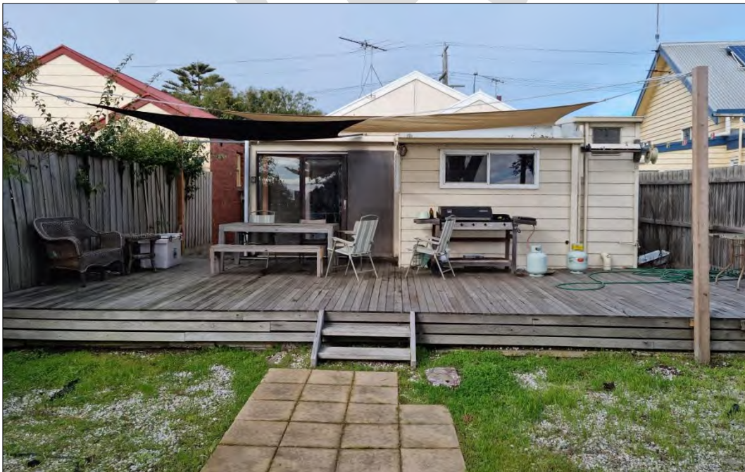
Rear view of 44 Wharf Street
