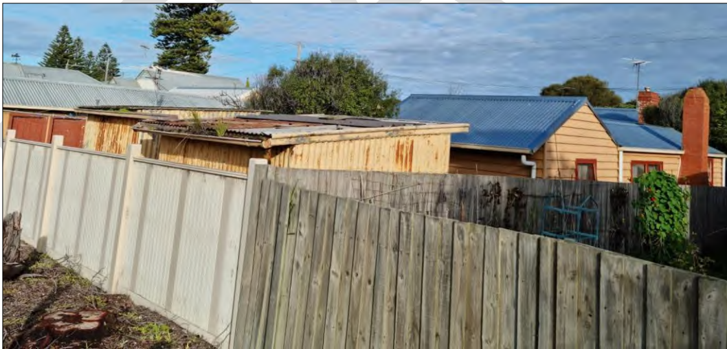
Rear view of 23 Beach Street, noting secondary cottages on right (brick chimney) and left (double wooden doors)
