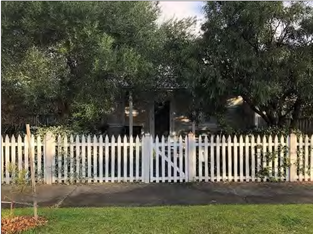
Street frontage of 34 Beach Street
