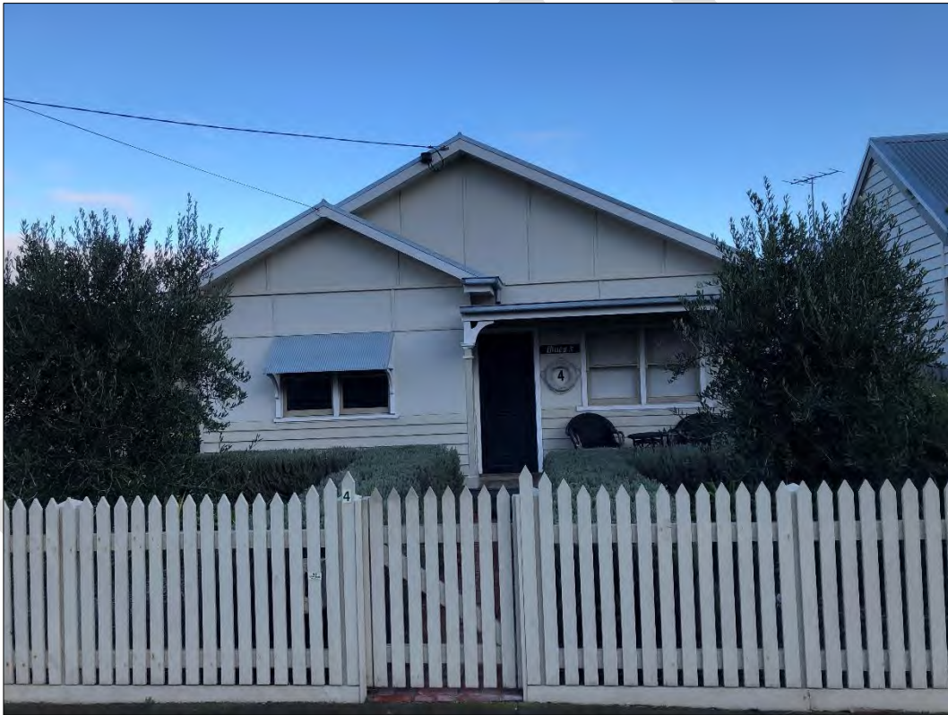
Street frontage of 4 Beach Street
