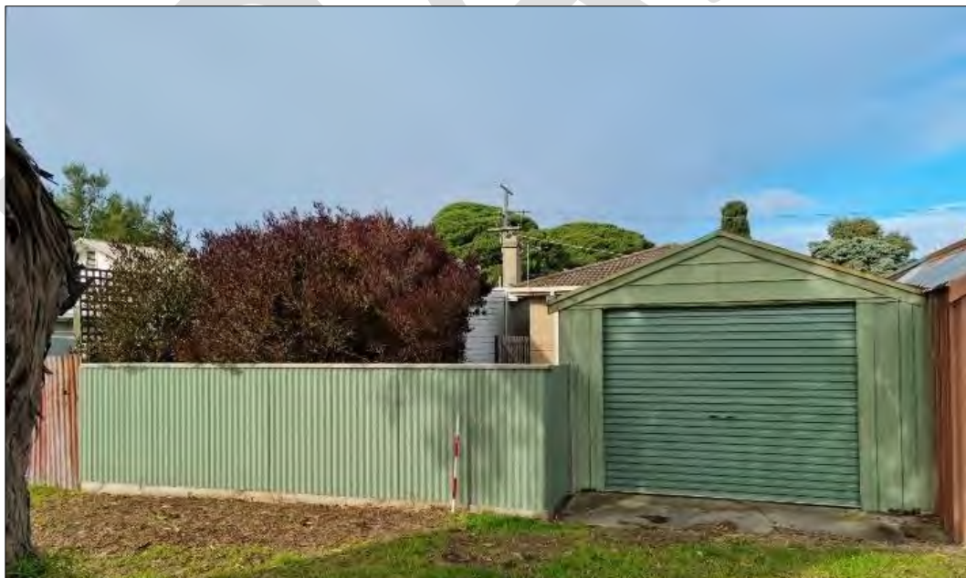
Rear view of 30 Wharf Street
