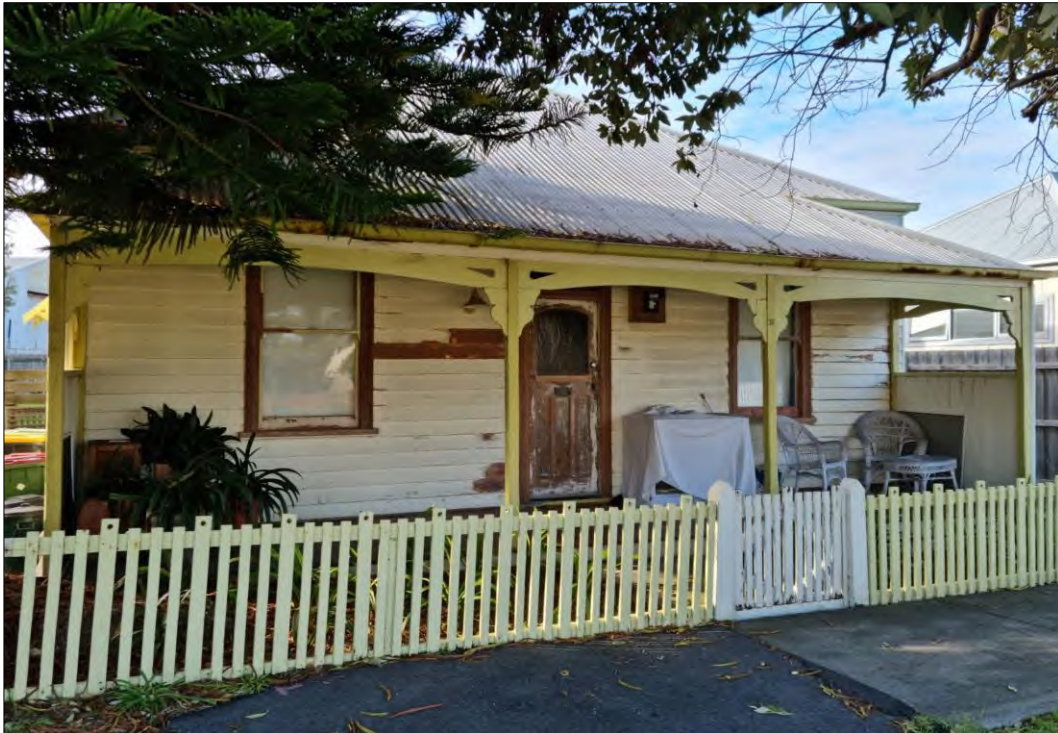
Street frontage of 35 Beach Street
