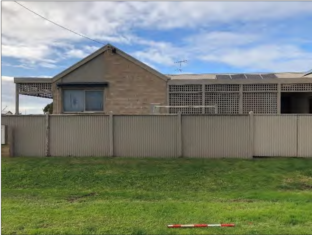
West-facing view of 1 Bridge Street
