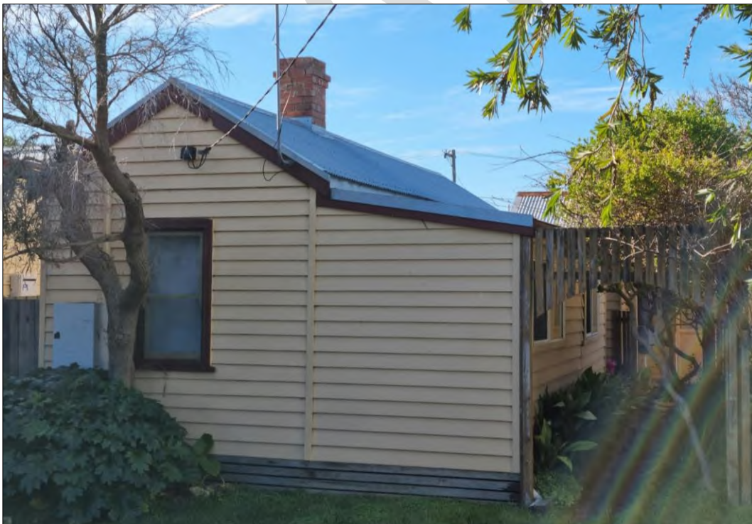
Weatherboard sleepout in rear of 16 Bay Street
