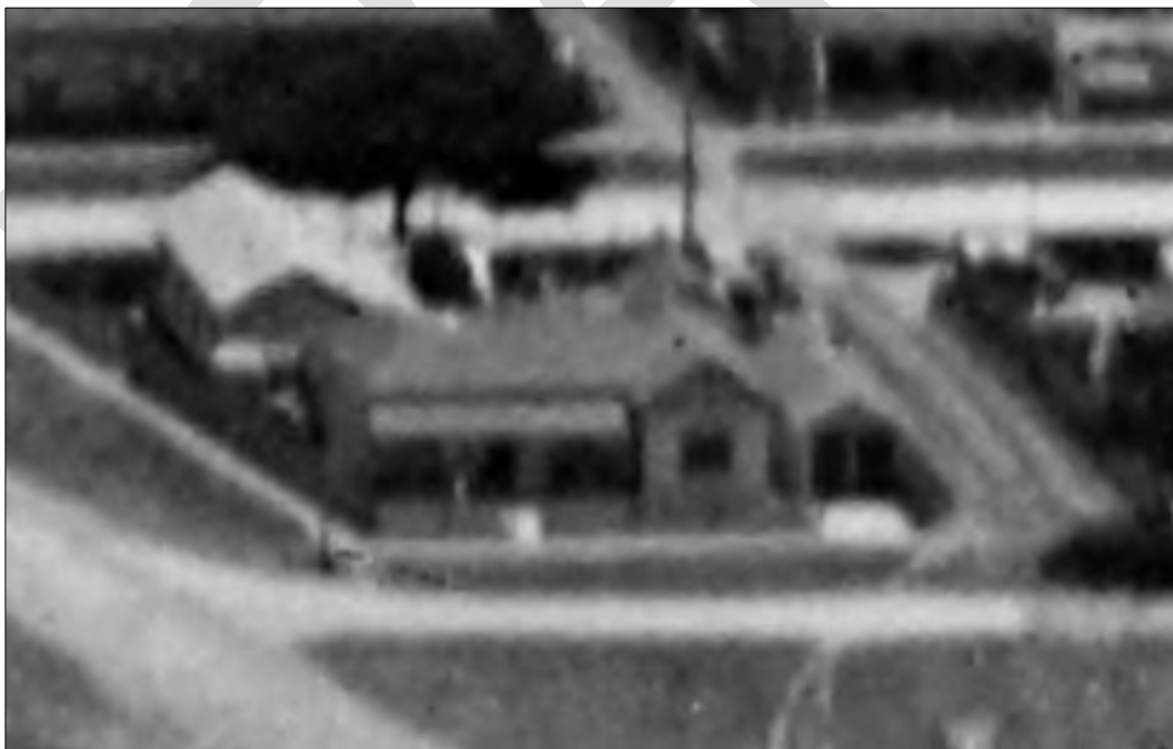
Aerial photograph of 6 Wharf Street dated 1928, showing original two houses and railway line behind property (Source: SLV 2023c). *Wharf Street running out of photograph on left.
