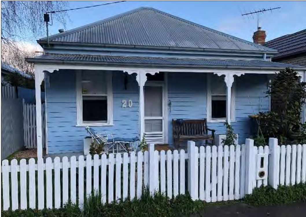
Street frontage of 20 Beach Street
