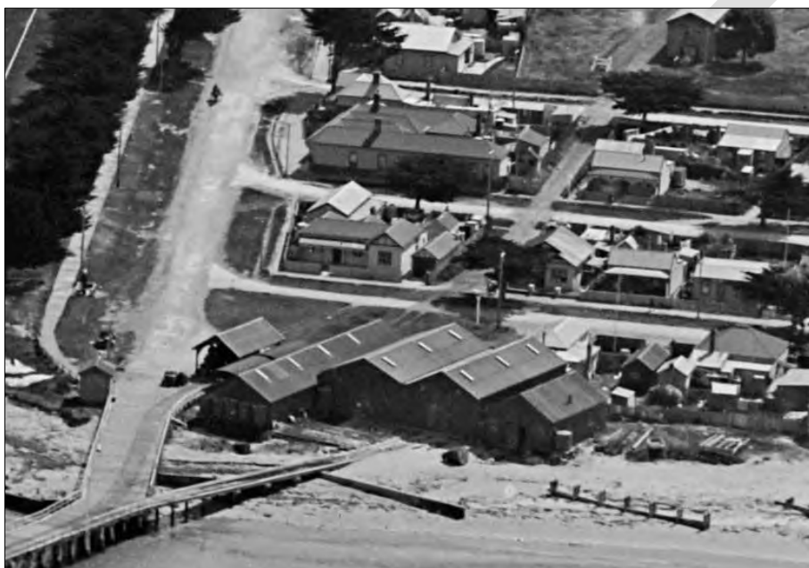
Figure 10: Former railway line to Fisherman's Pier (foreground), traversing behind Wharf Street properties, dated 1928 (Source: SLV 2023c).
