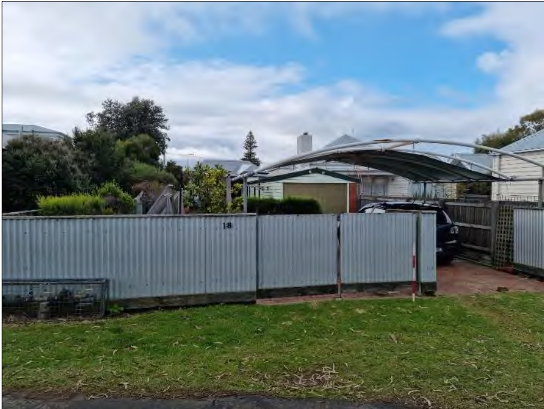
Rear view of 18 Bridge Street
