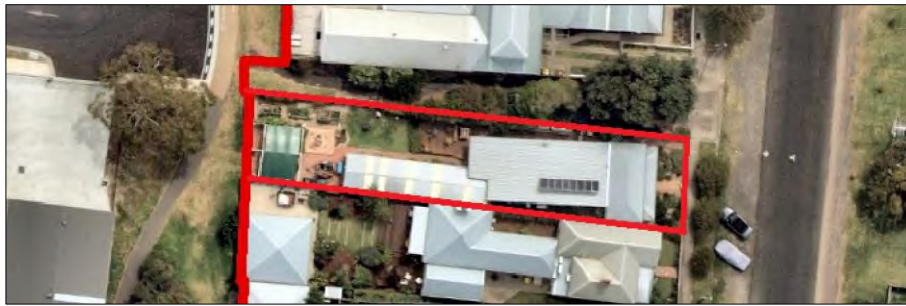
Aerial view of 18 Bridge Street (Source: Nearthmap)
