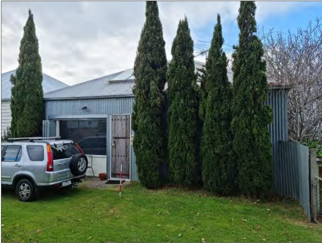
Rear view of 22 Bridge Street
