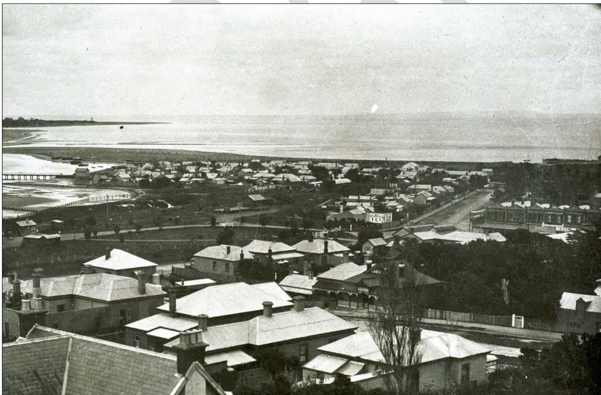
Figure 7: Photograph looking north-east over Fisherman's Flat, dated c.1910 (Source: Queenscliff Historical Museum (QHM) 2023).
