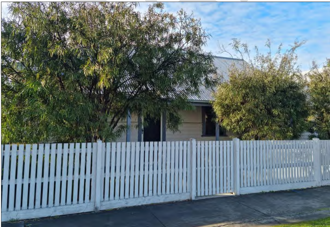
Street frontage of 37 Beach Street
