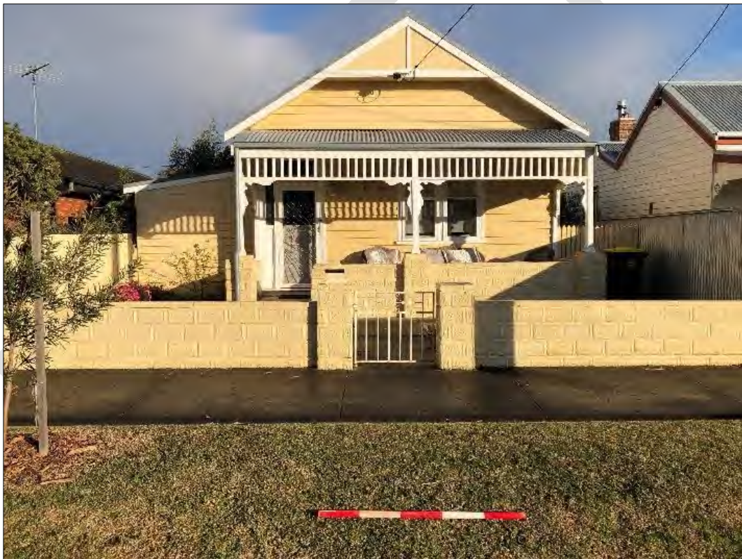
Street frontage of 28 Beach Street
