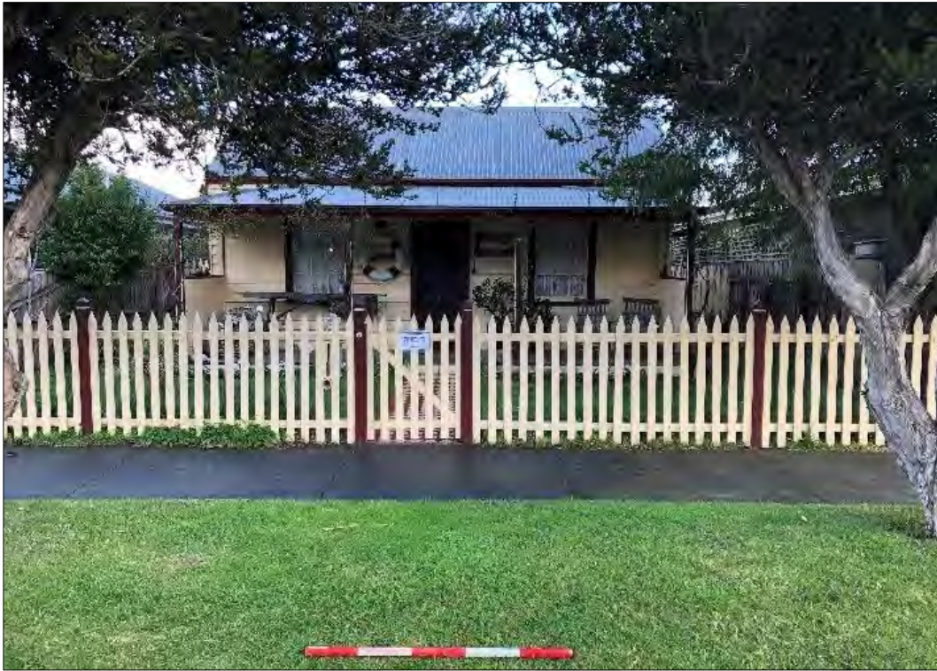
Street frontage of 12 Beach Street
