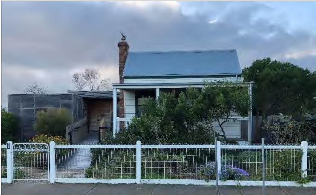
Street frontage of 11 Beach Street
