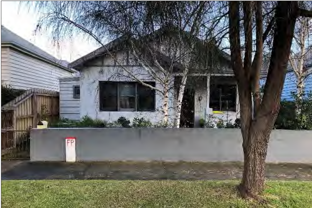
Street frontage of 22 Beach Street
