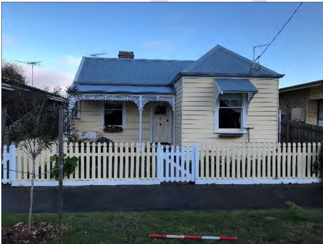
Street frontage of 8 Beach Street
