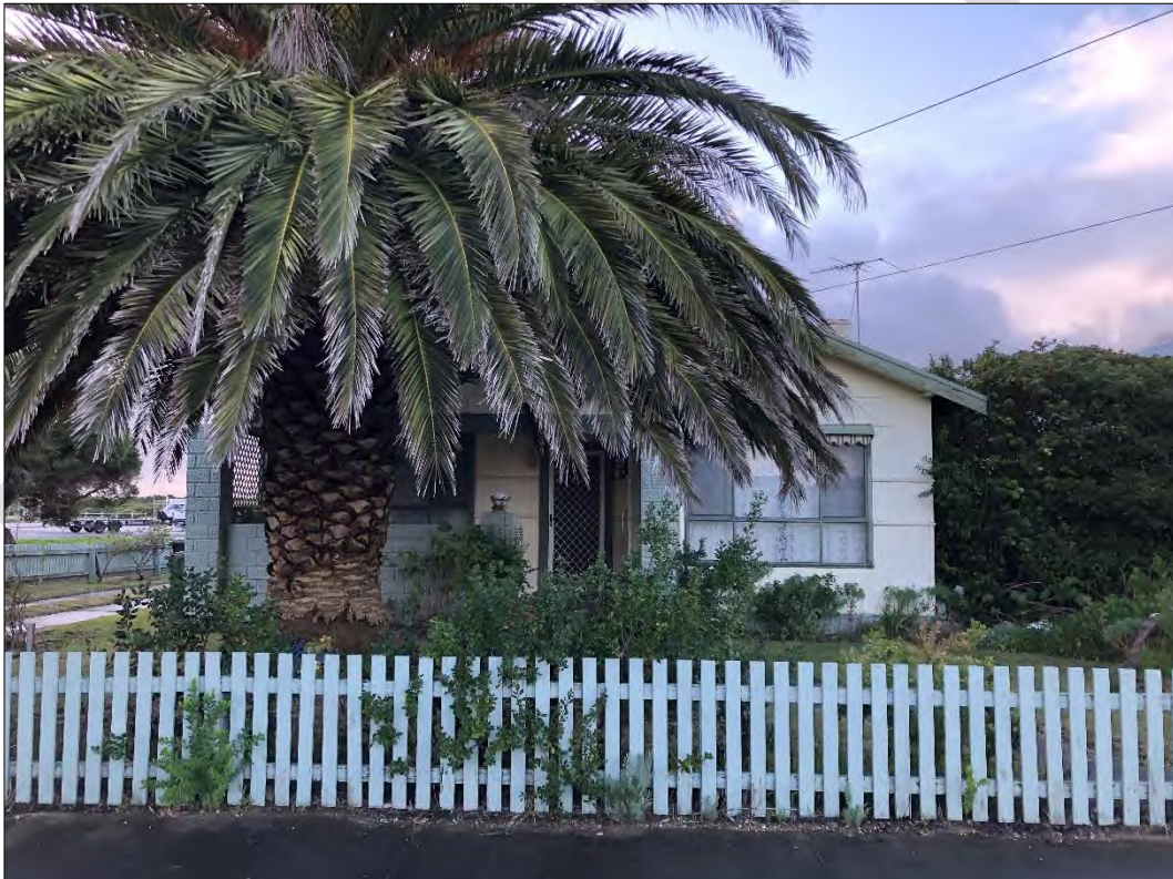
Street frontage of 5 Beach Street
