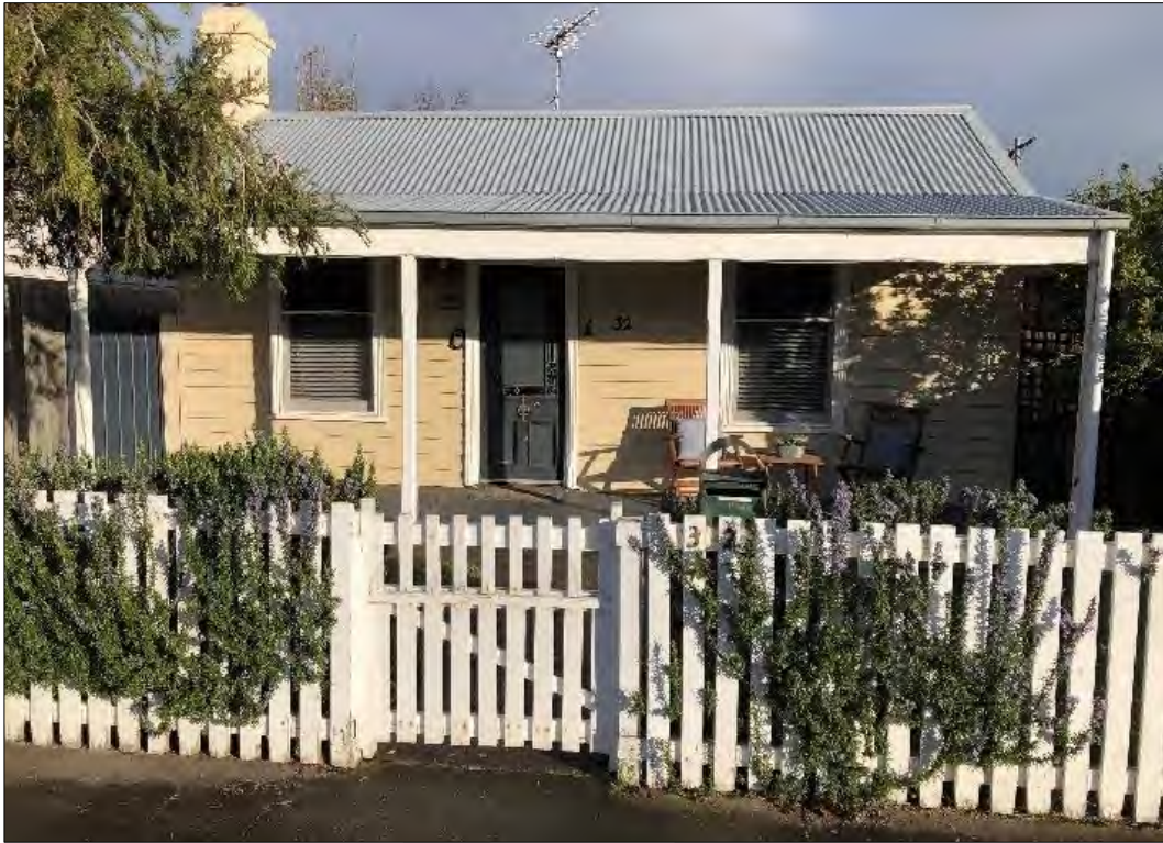
Street frontage of 32 Beach Street
