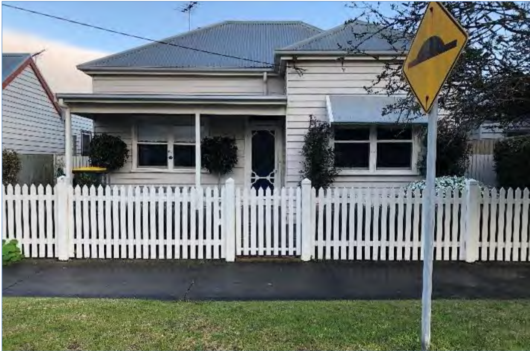
Street frontage of 24 Beach Street
