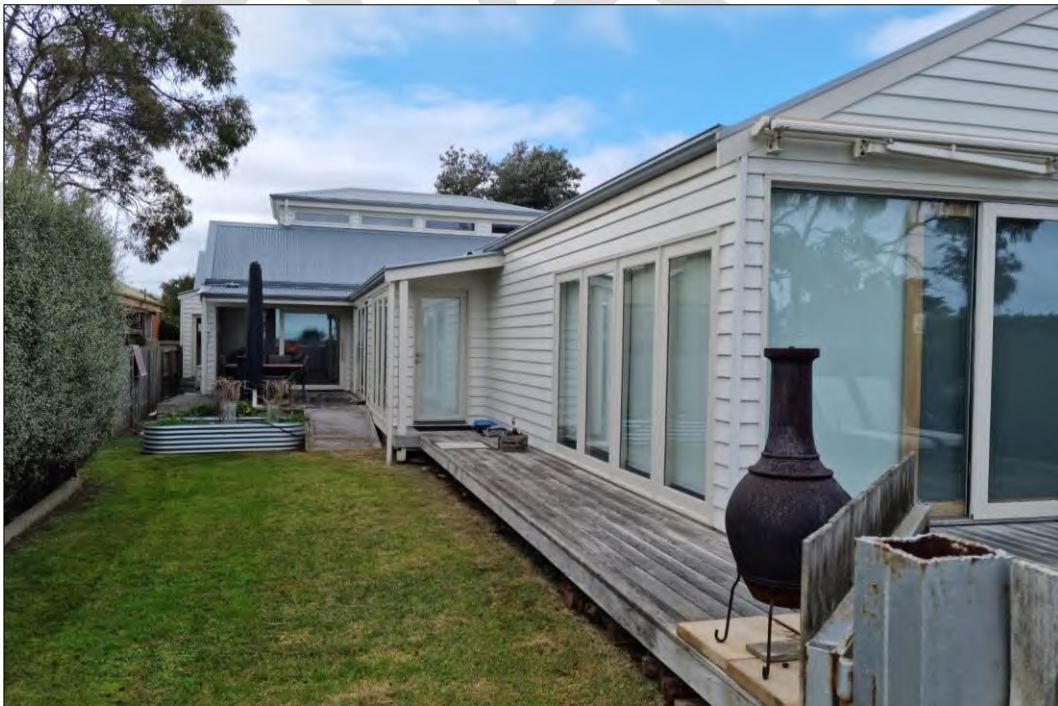
Rear view of 16 Bridge Street
