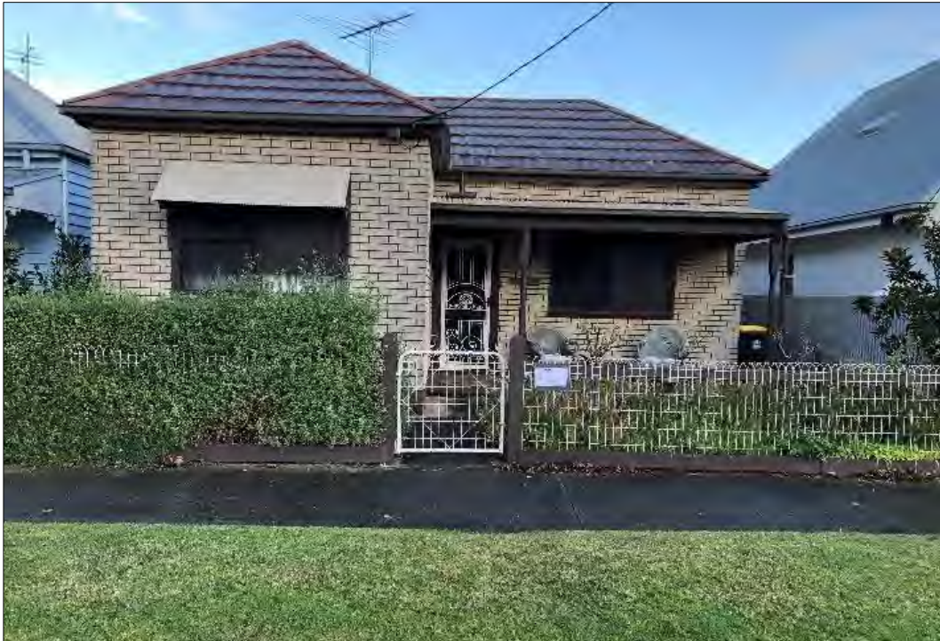
Street frontage of 18 Beach Street
