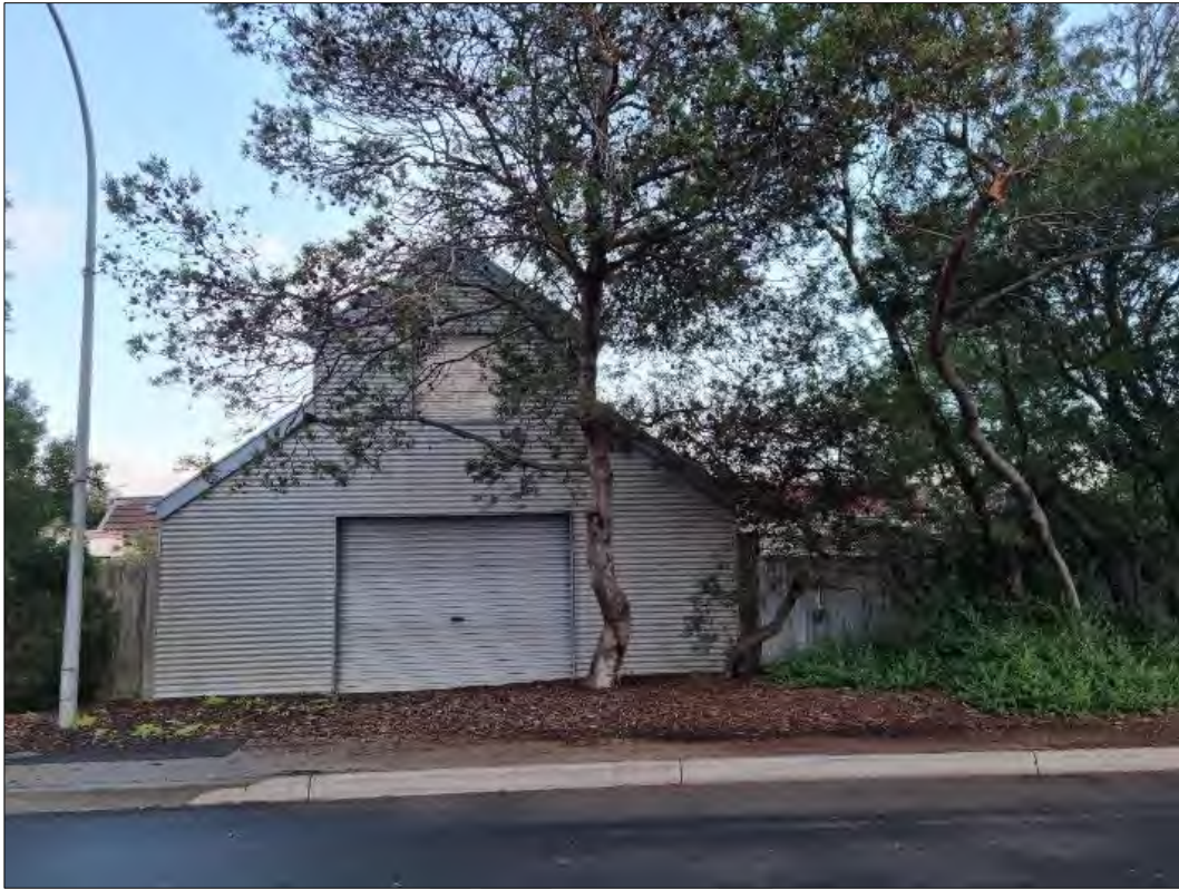
Two-storey garage facing Harbour Street
