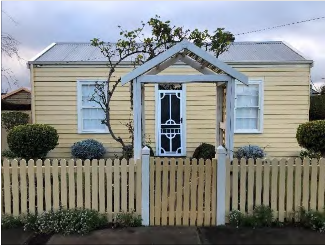
Street frontage of 27 Beach Street
