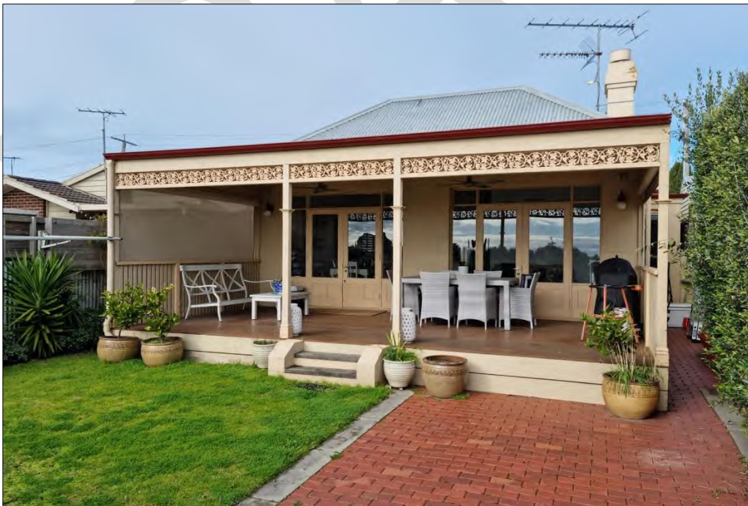
Rear view of 34 Wharf Street
