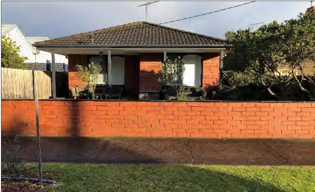
Street frontage of 30 Beach Street
