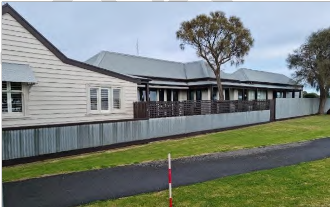
North-facing view of 6 Bridge Street
