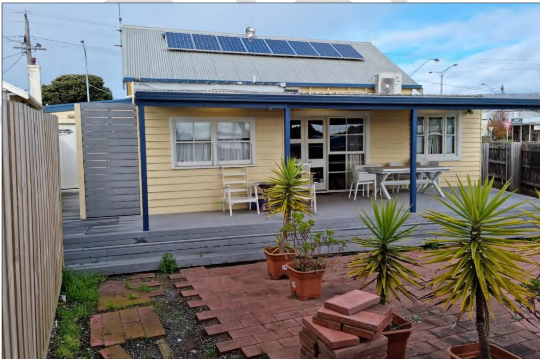
Rear view of 46 Wharf Street
