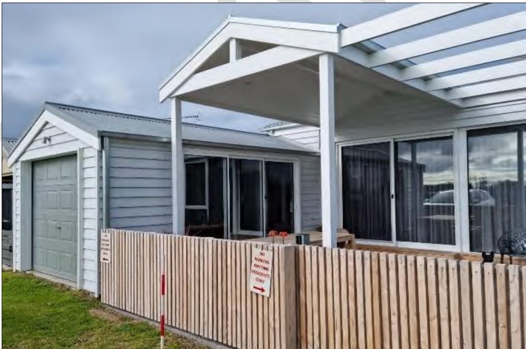
Rear view of 38 Wharf Street
