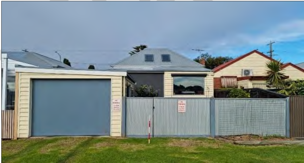
Rear view of 40 Wharf Street
