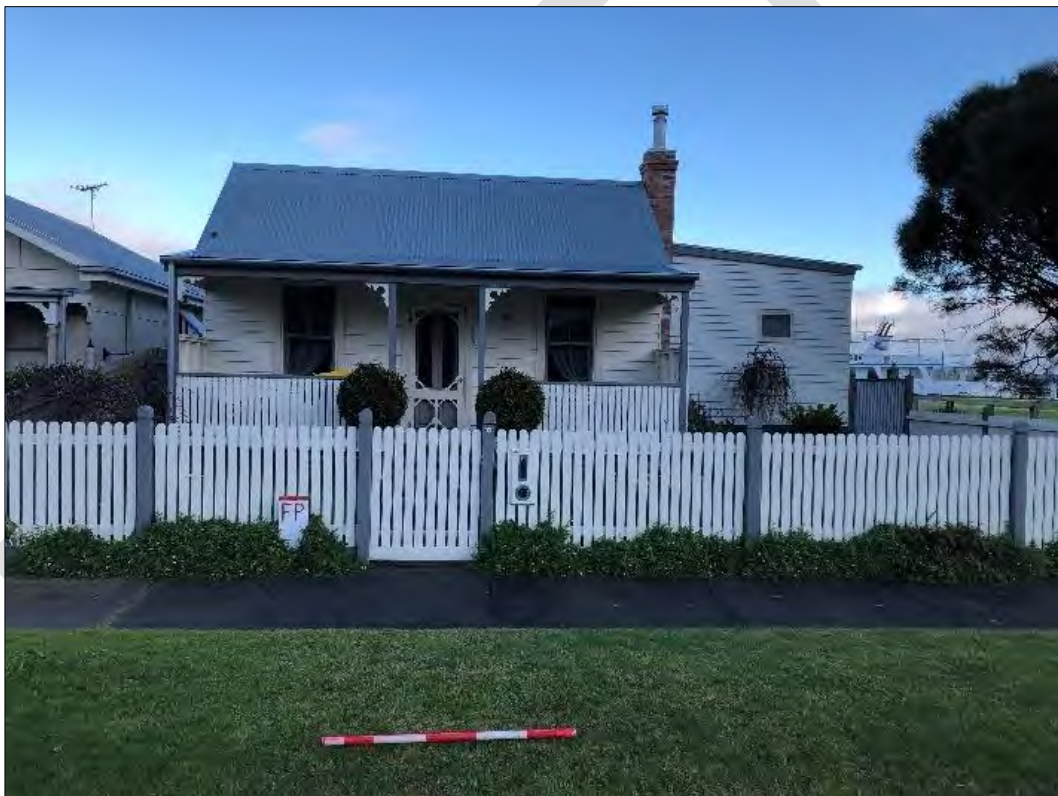
Street frontage of 2 Beach Street
