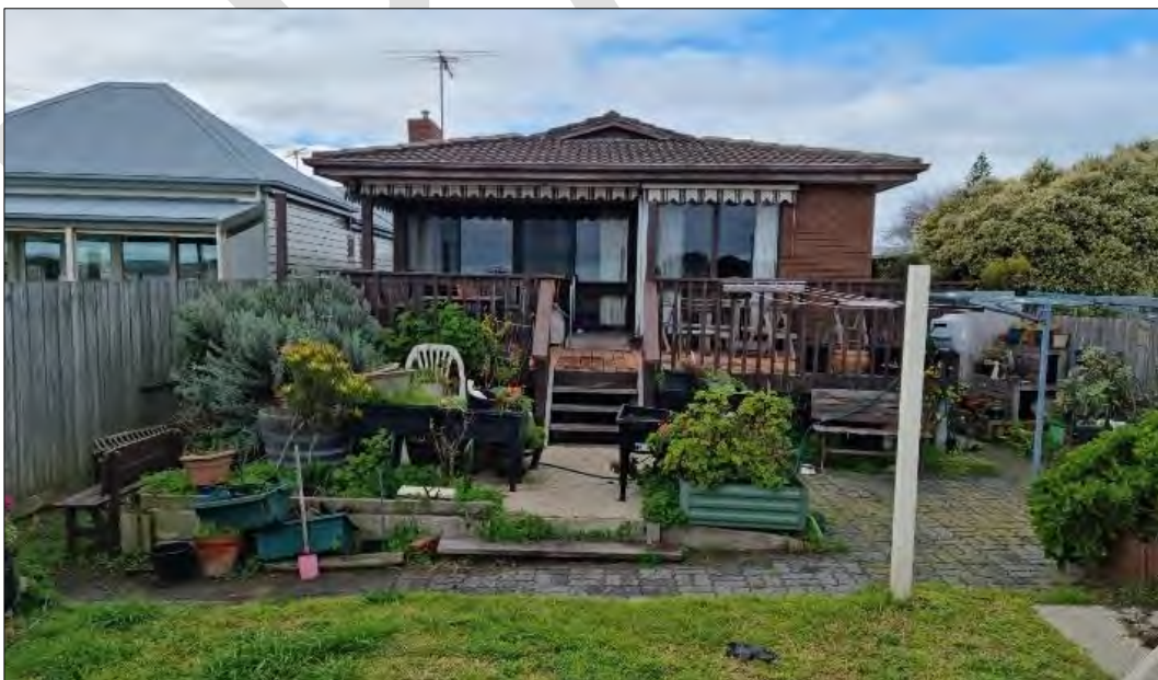
Rear view of 10 Bridge Street
