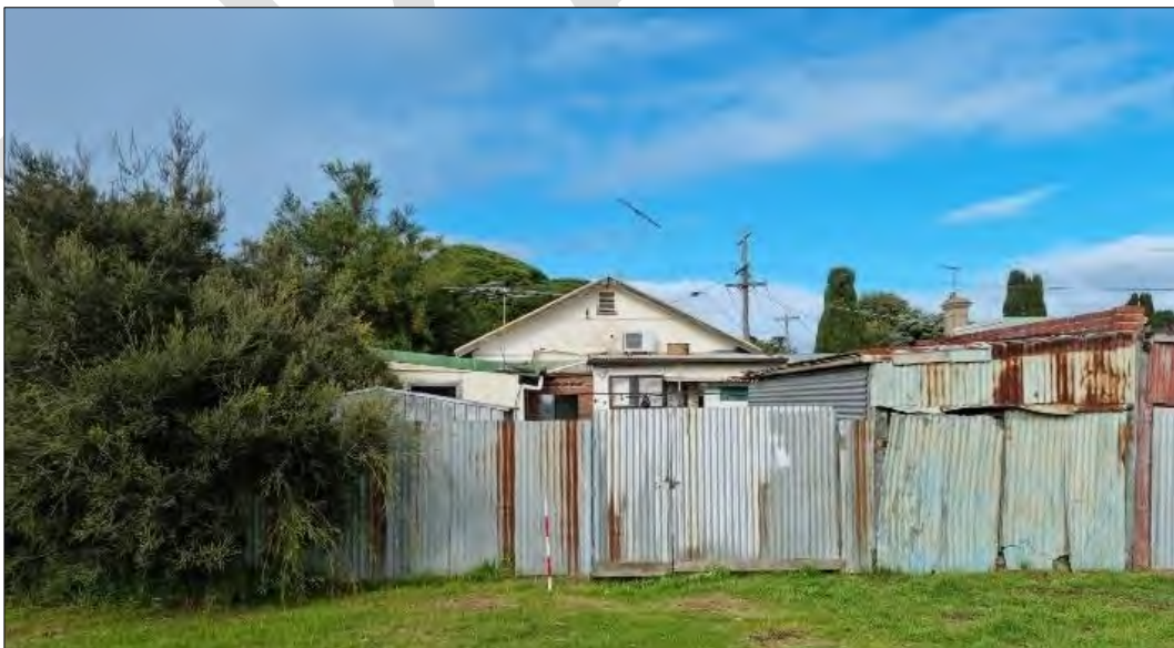
Rear view of 26 Wharf Street
