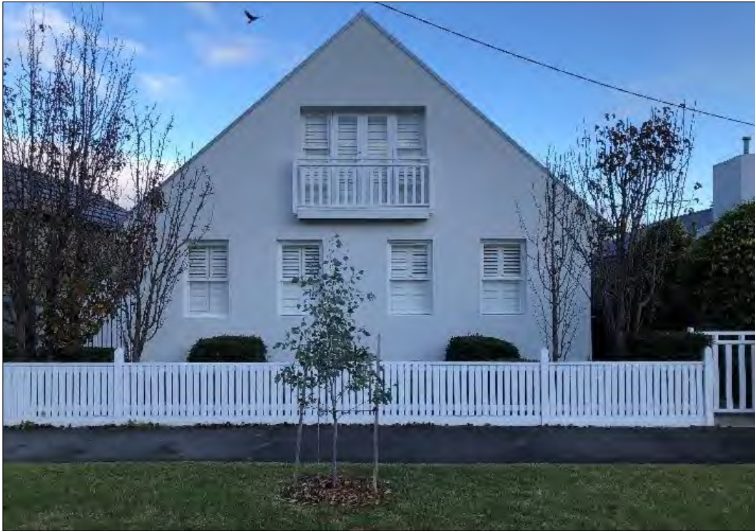
Street frontage of 16 Beach Street
