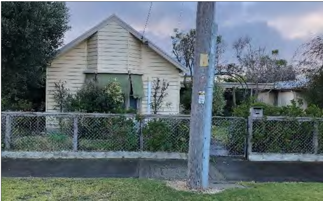
Street frontage of 9 Beach Street
