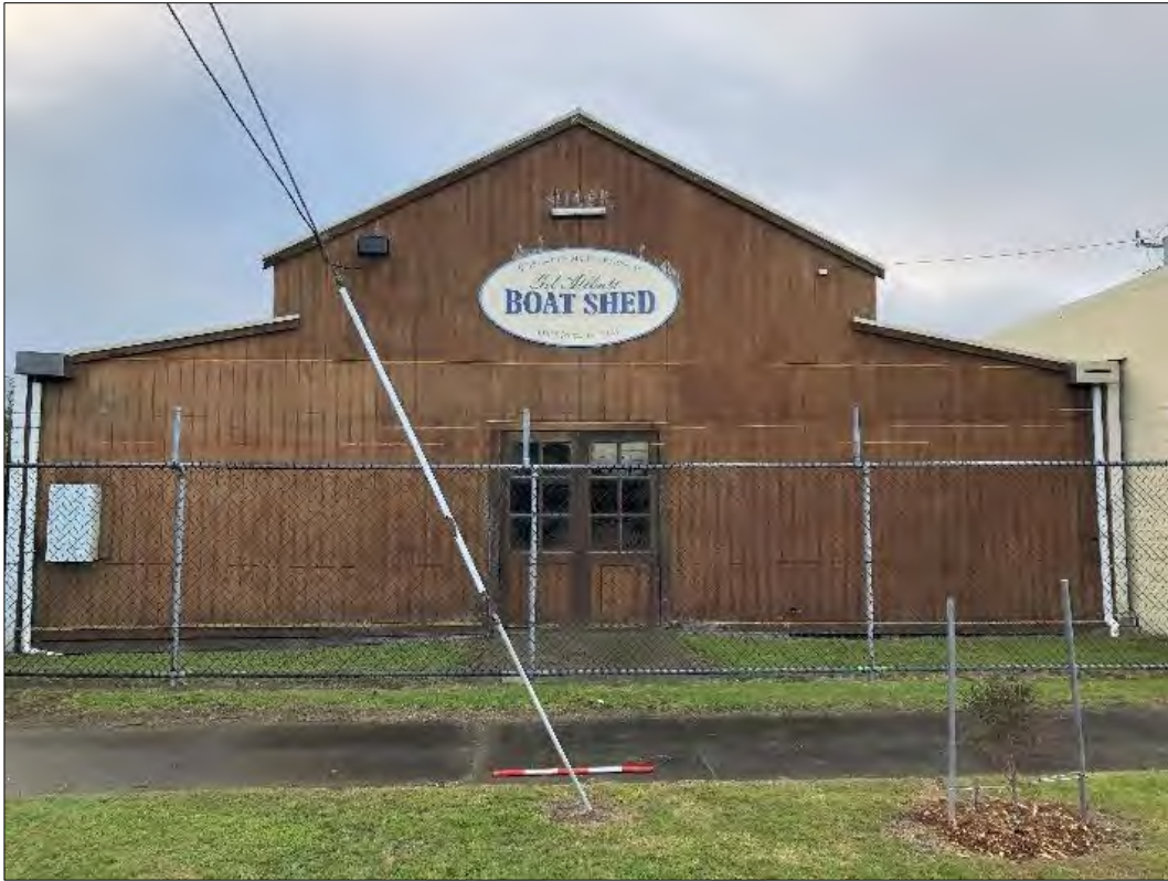
Street frontage of 39 Beach Street
