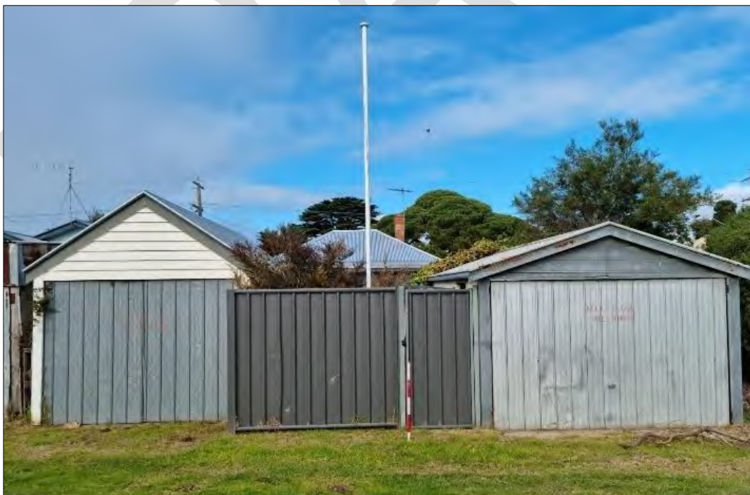
Rear view of 22 Wharf Street
